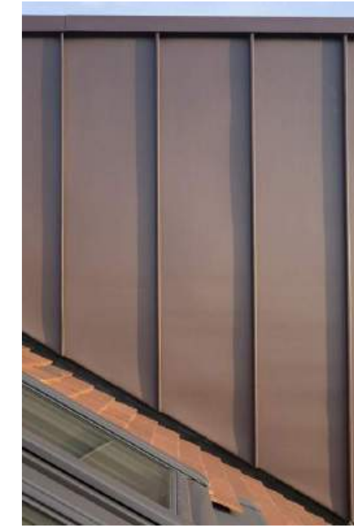
REFINISHED METAL ROOF
