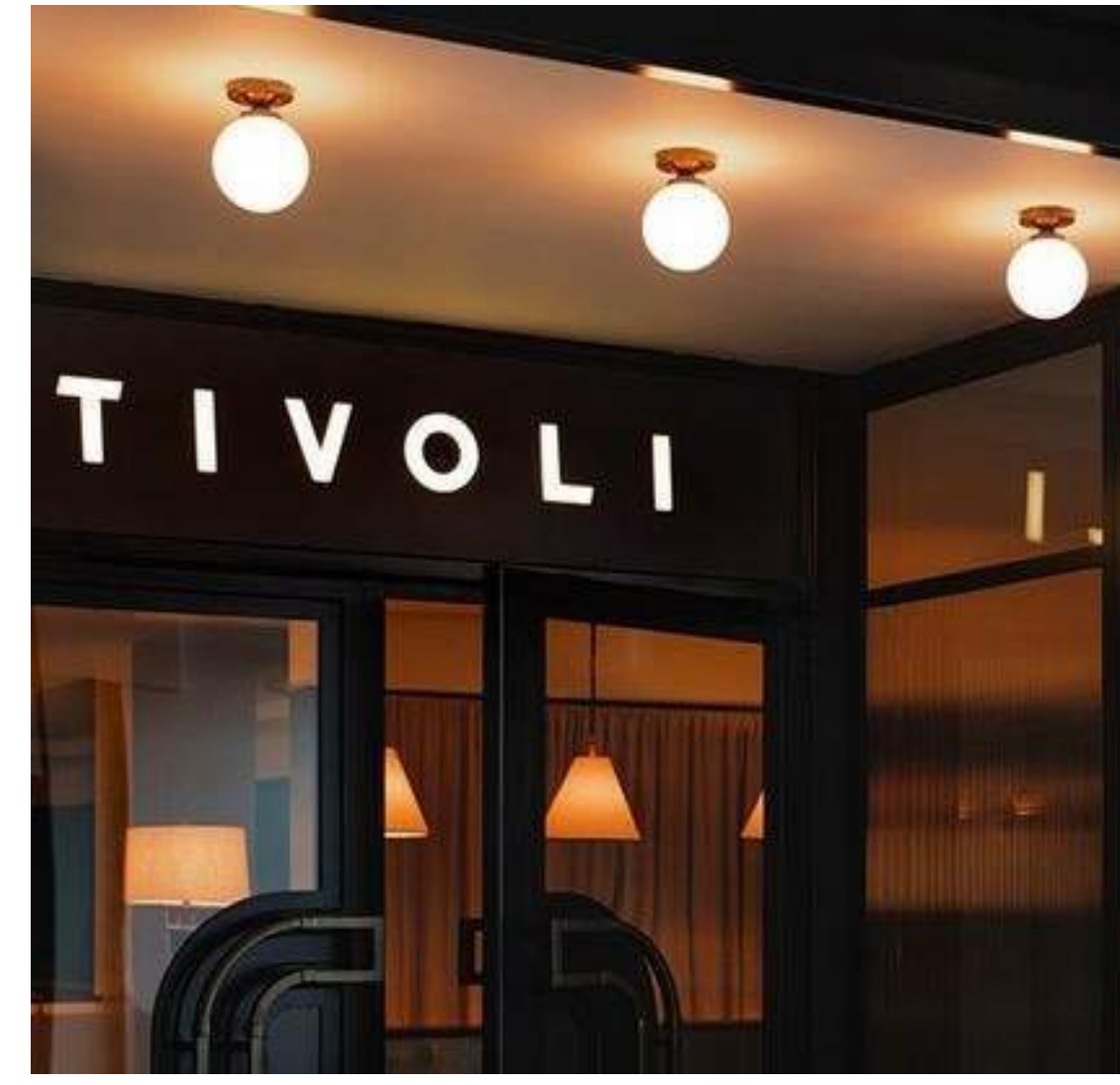
TINTED GLASS MEDIUM - DARK TINT AT MAIN ENTRY STOREFRONT
