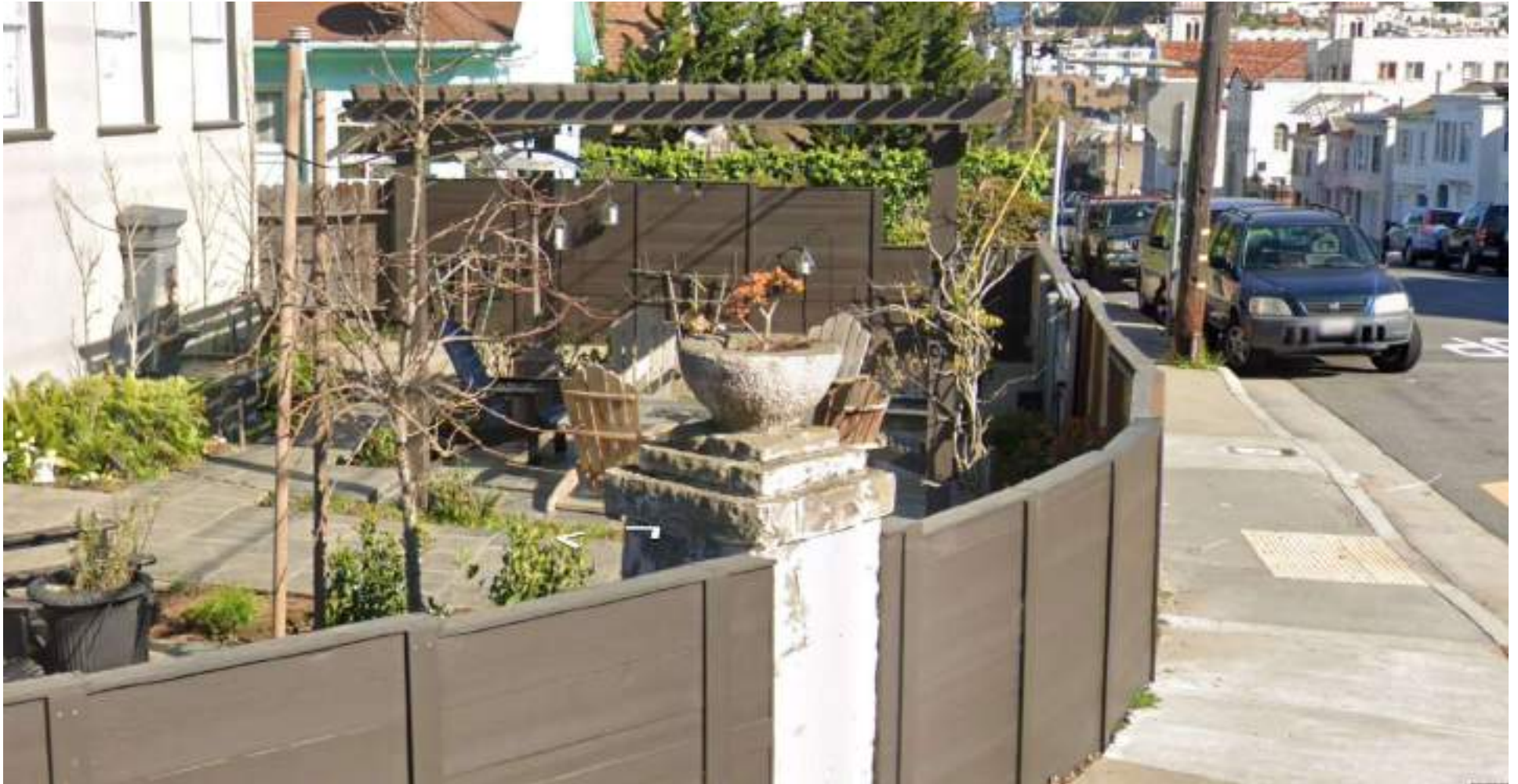
Portions of the pergola, gas fire table, landscaping, special pavers, and fence encroaching onto Ashton Ave.
