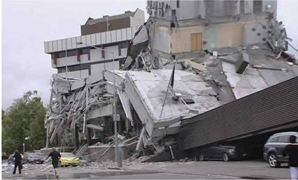
Damage to CTV building following Christchurch earthquake. Source: 1 NEWS
