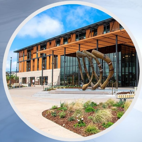
Southeast Community Center
