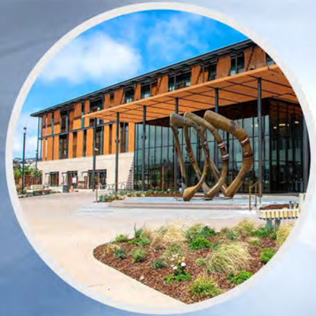
Southeast Community Center
