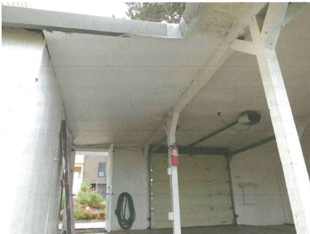
Figure 2: 617 Sanchez Street, front carport, interior
