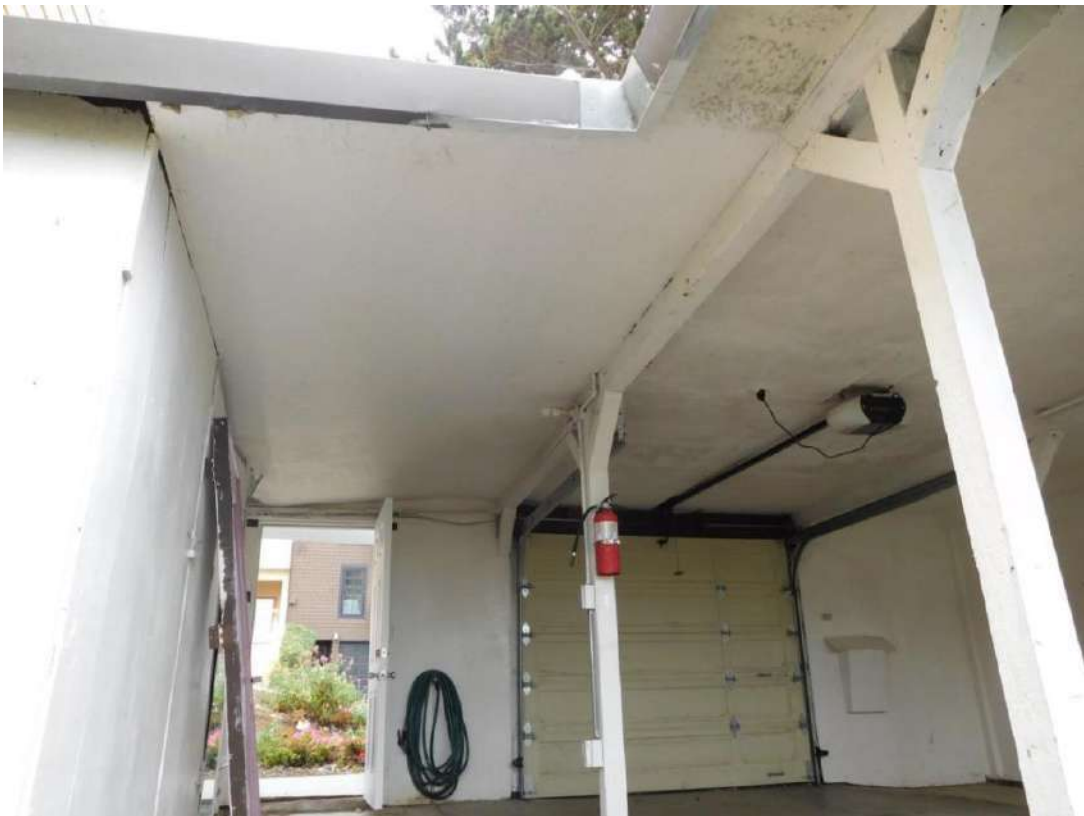
Figure 2: 617 Sanchez Street, front carport, interior
