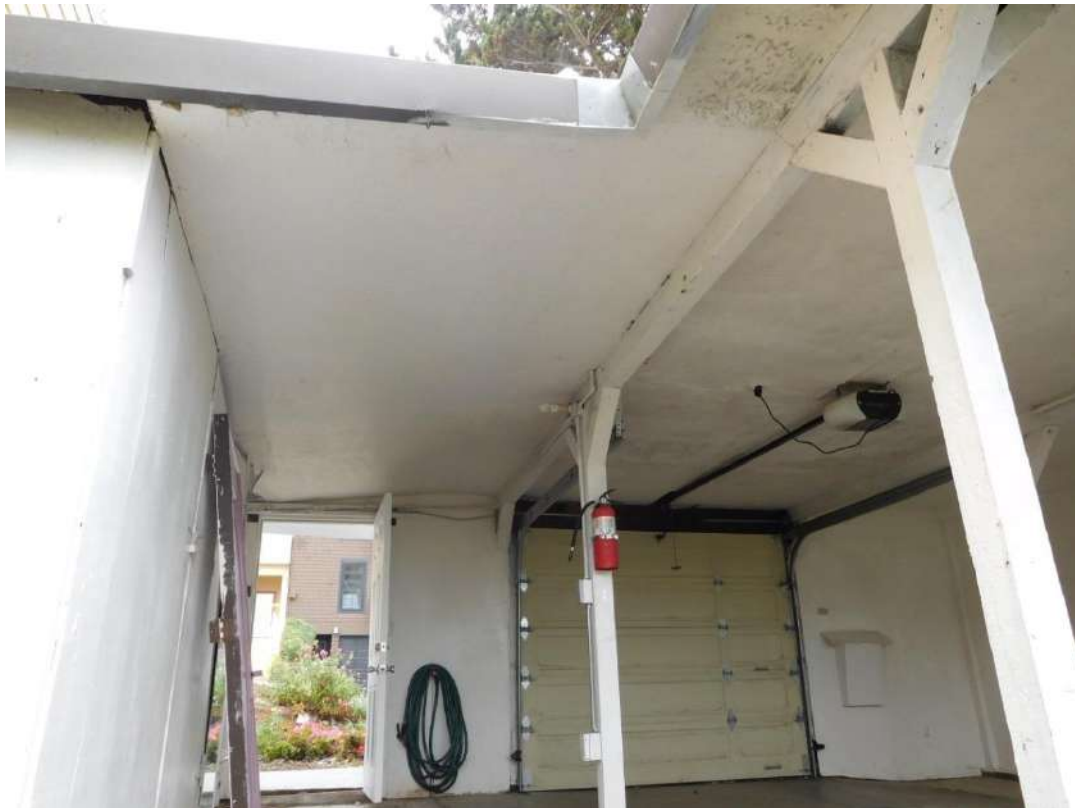
Figure 2: 617 Sanchez Street, front carport, interior
