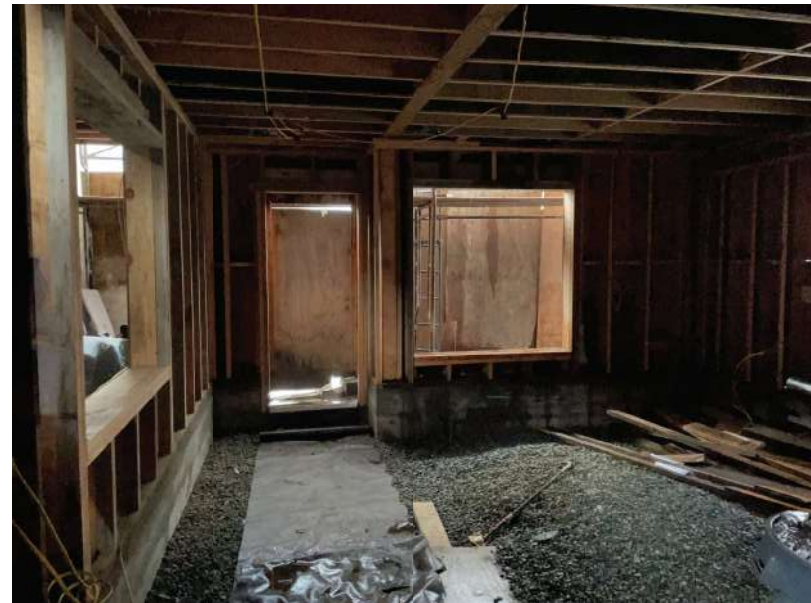
① 1ST LEVEL, AS BUILT REAR CONDITION (03/2023) SCALE: 1/8" = 1'-0"
