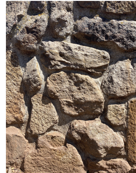
STONES FROM EXISTING BENCHES
