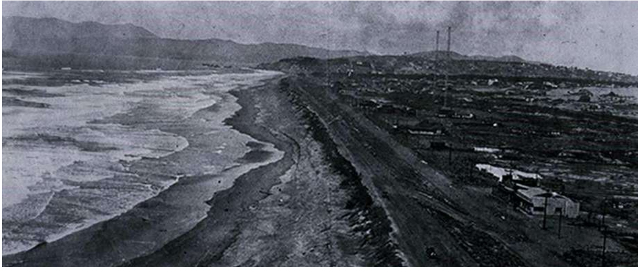
Embankment constructed for the Great Highway near Pacheco Street, 1915. Note the shore embayment characteristic of this location, where a seawall was constructed in the 1990s. (Olmsted & Olmsted, 1979).
