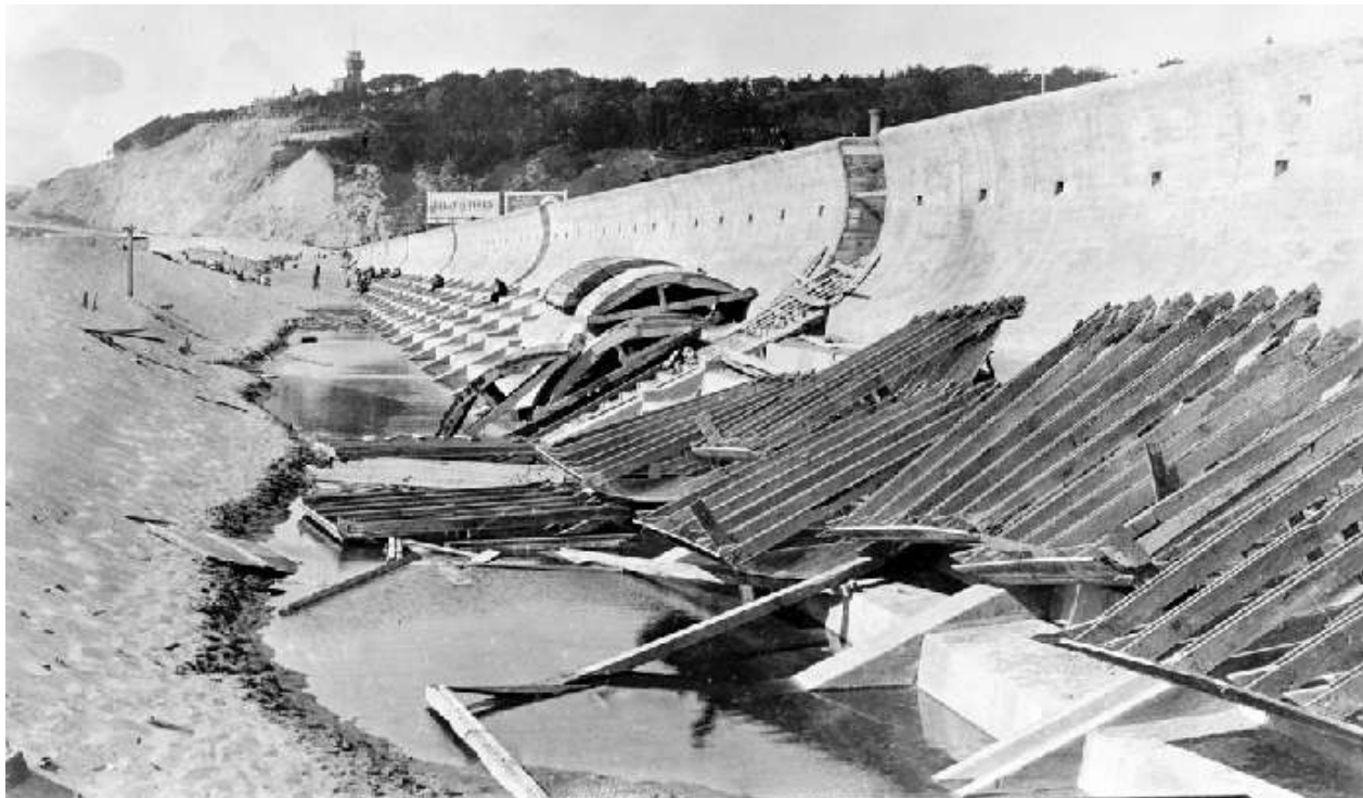
View north from foot of Cabrillo St during the second phase of construction of the O'Shaughnessy Seawall. Photo from August 1922. Source: Western Neighborhoods Project - wnp36.02888.
