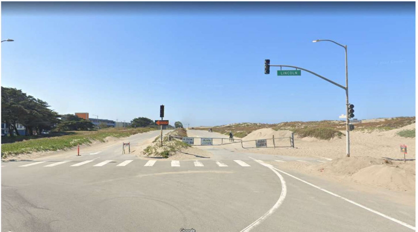
GREAT HIGHWAY AT LINCOLN WAY (looking south)
