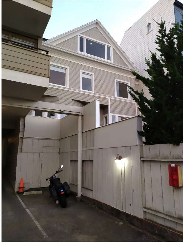
2020 Photo - NO TRASH ENCLOSURE
