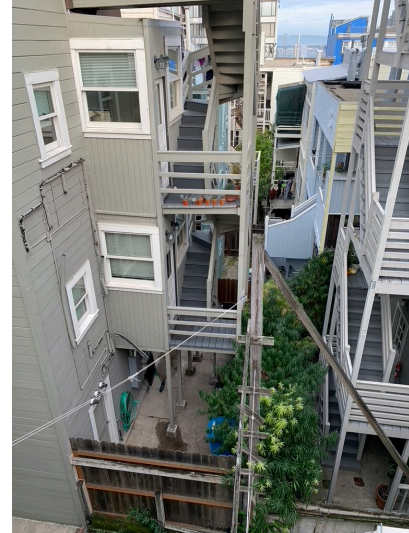
Figure 4. The tenement-like situation immediately east of 45-49 Bernard Street.
