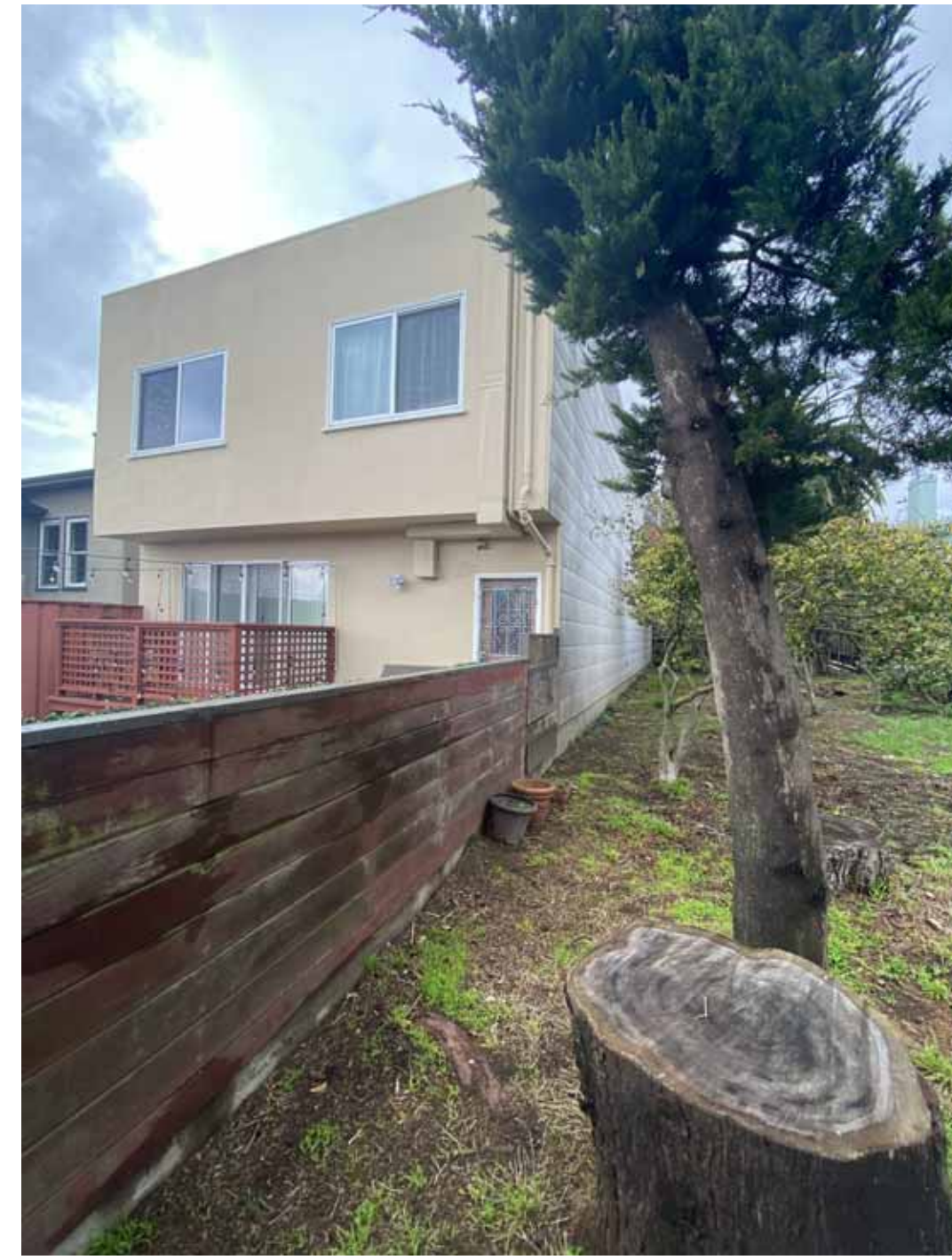
ADJACENT PRTY. 35 SANTA ROSA ST REAR VIEW
