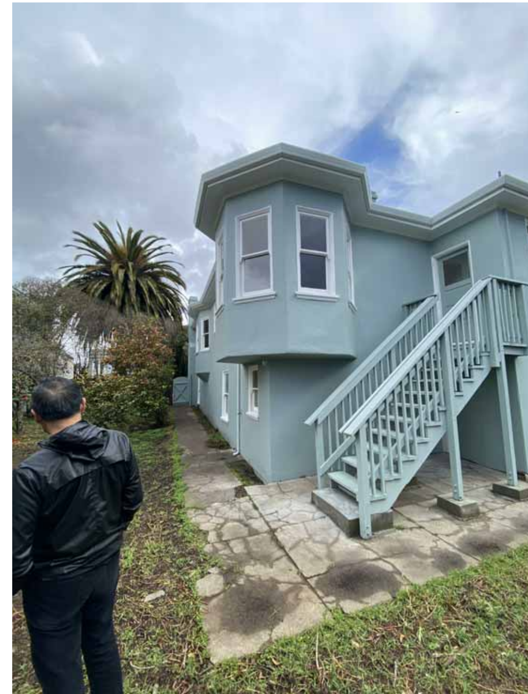
ADJACENT PRTY. 25 SANTA ROSA ST REAR VIEW
