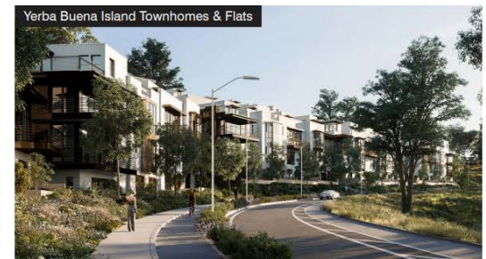
31 Townhomes and Condos, Under Construction
