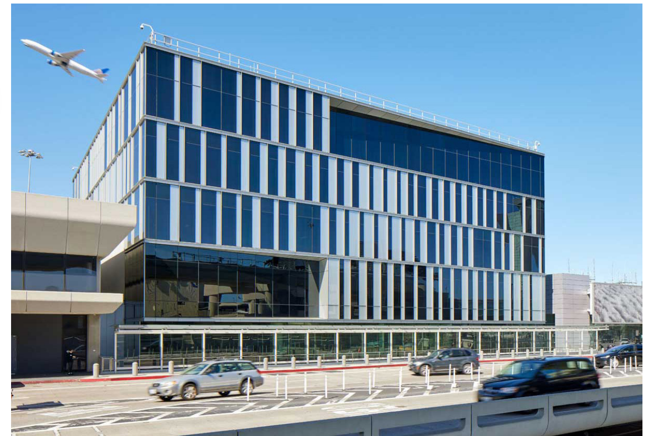
B. EXISTING COURTYARD 3 BUILDING
