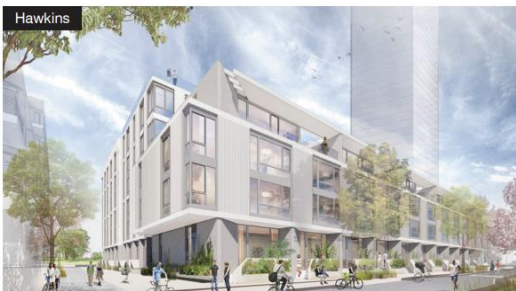
178 Apartments, Under Construction
