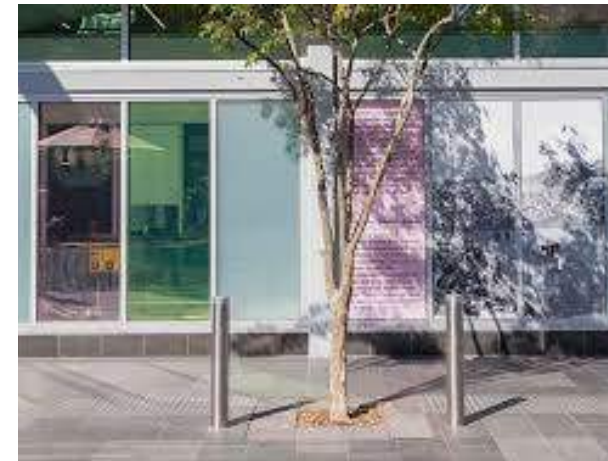
Bollard Protection at Trees
