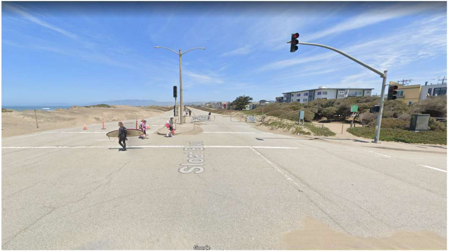
GREAT HIGHWAY AT SLOAT BOULEVARD (looking north)
