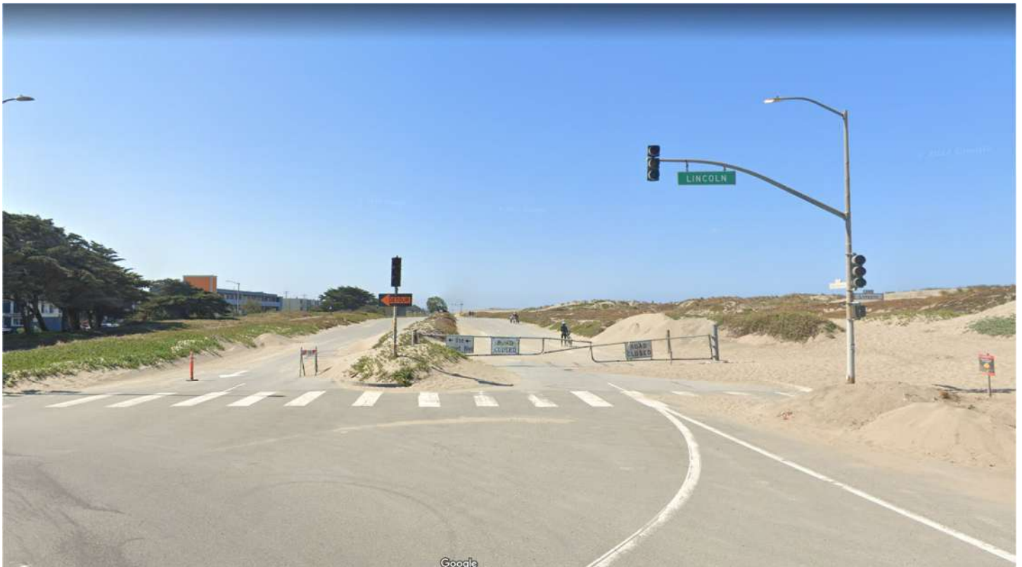
GREAT HIGHWAY AT LINCOLN WAY (looking south)
