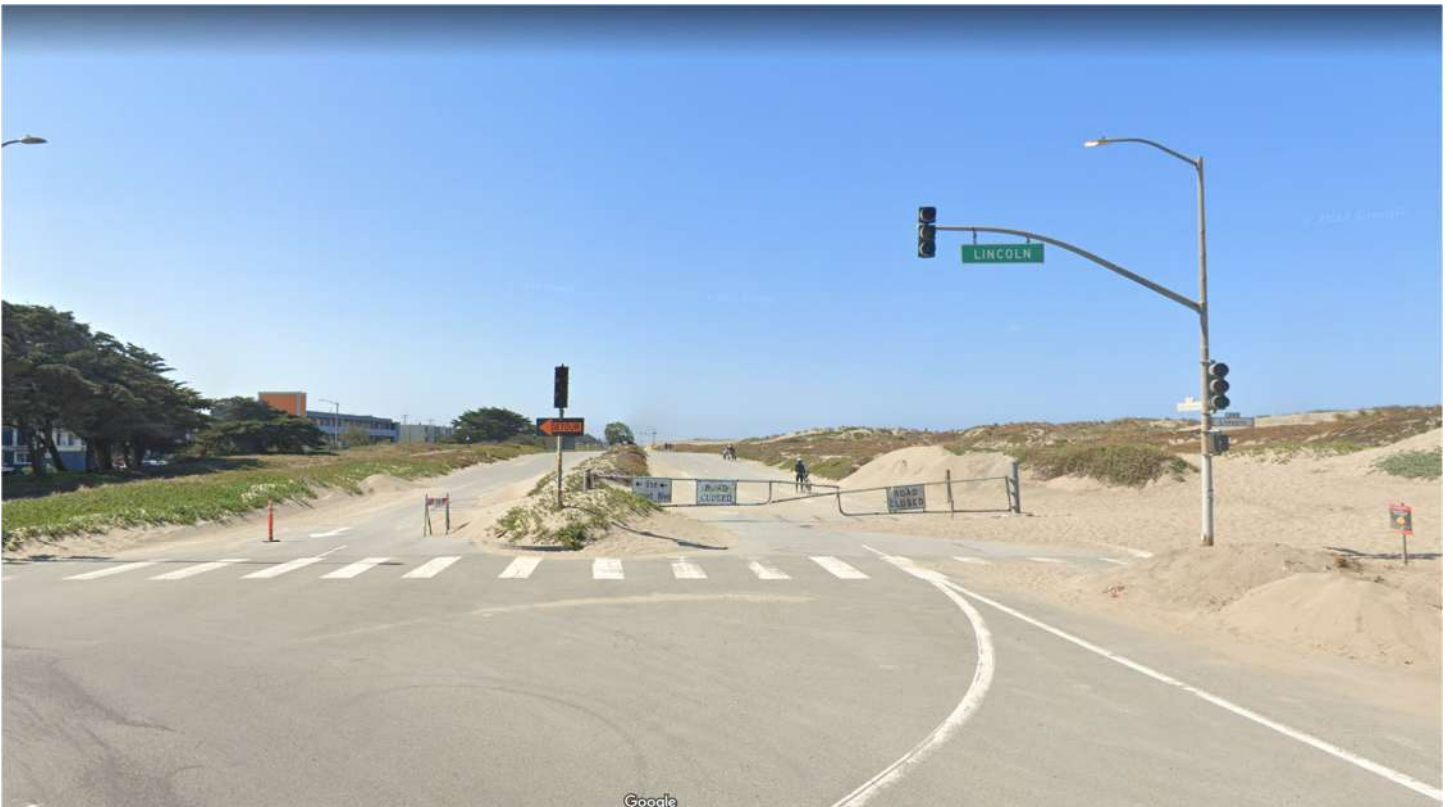
GREAT HIGHWAY AT LINCOLN WAY (looking south)
