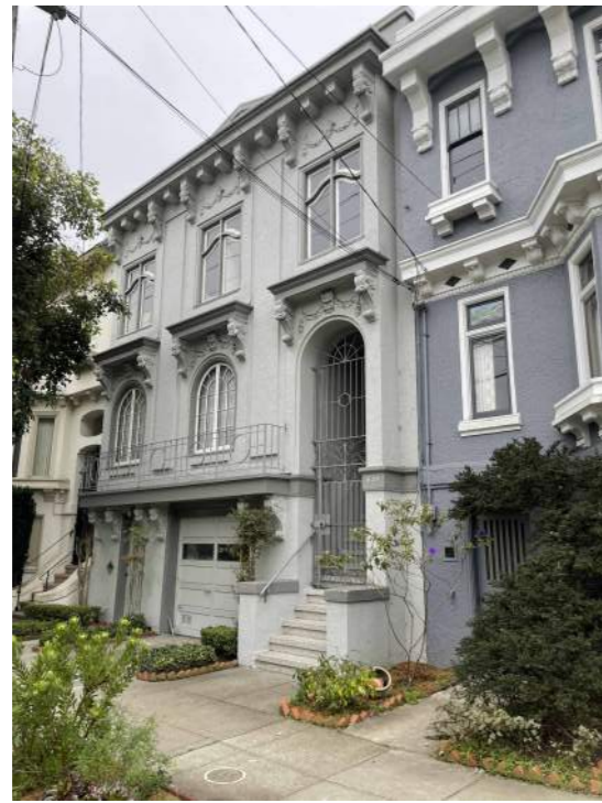
(F) FRONT FACADE OF SUBJECT BUILDING
