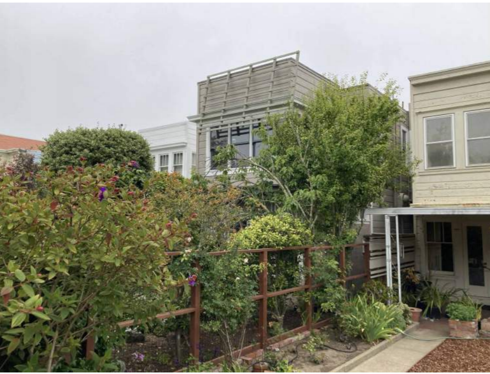
(D) REAR VIEW OF THE ADJACENT BUILDING (679 12th AVENUE)
