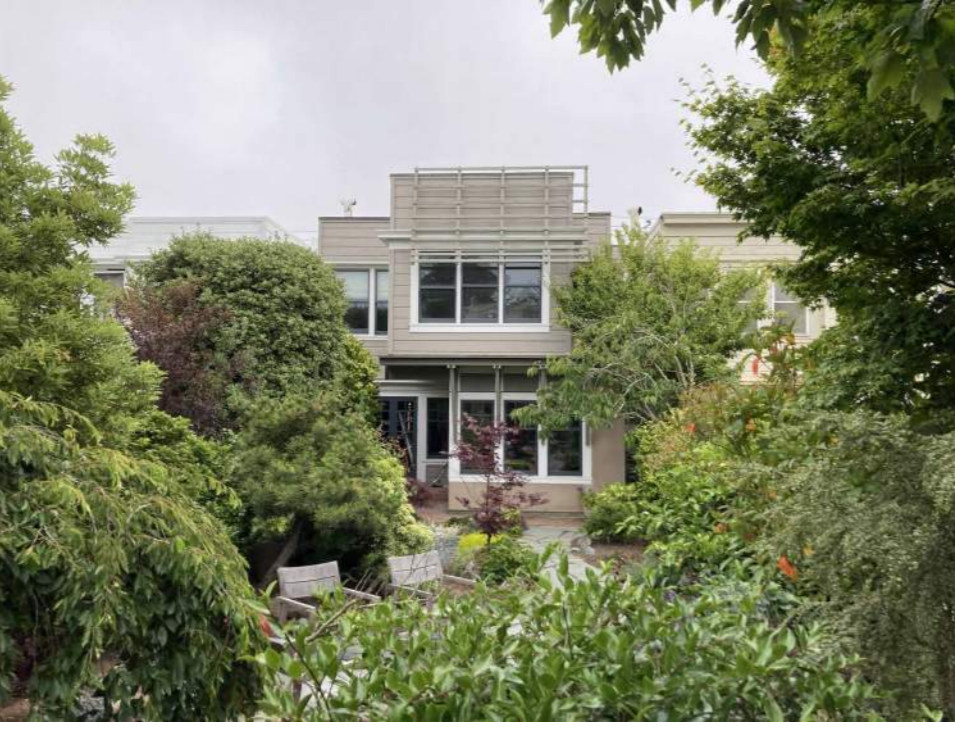
(B) REAR VIEW OF THE ADJACENT BUILDING (679 12th AVENUE)
