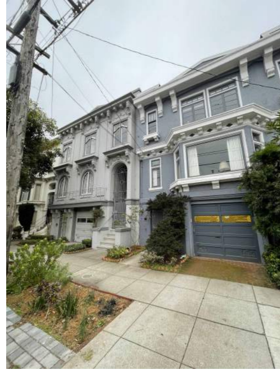
(G) FRONT FACADE OF ADJACENT BUILDING (679 12th AVENUE)
