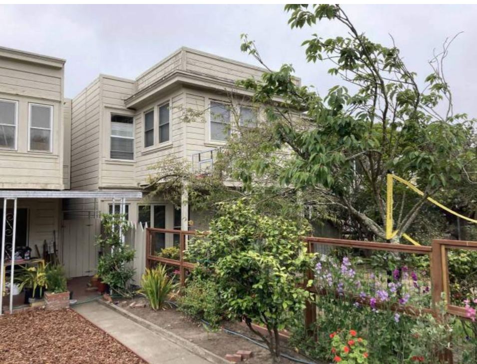
(E) REAR VIEW OF THE ADJACENT BUILDING (683 12th AVENUE)
