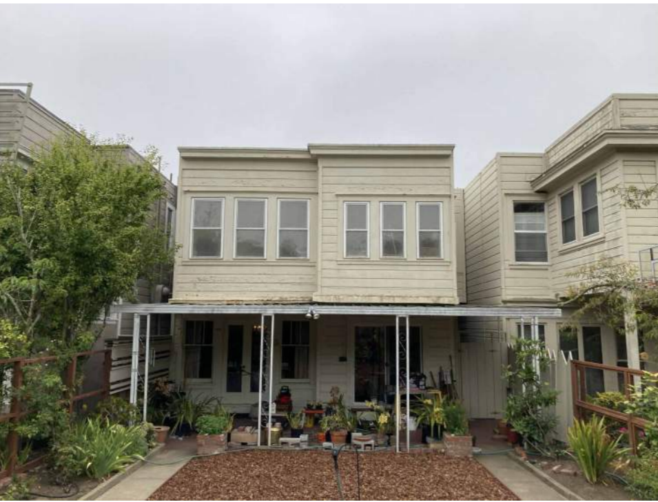
(A) REAR FACADE OF THE SUBJECT BUILDING
