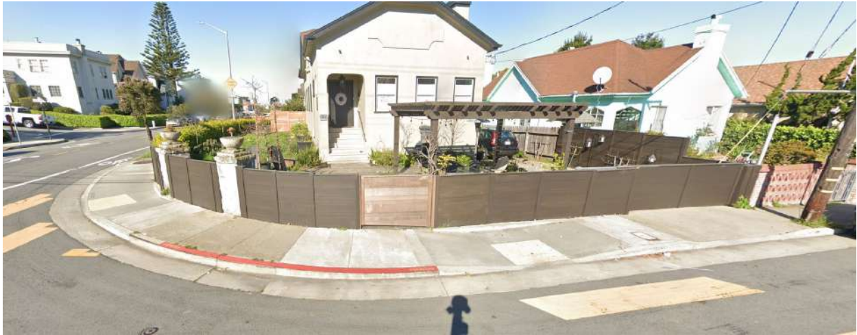
Figure 2. Non-standard curb ramp.
