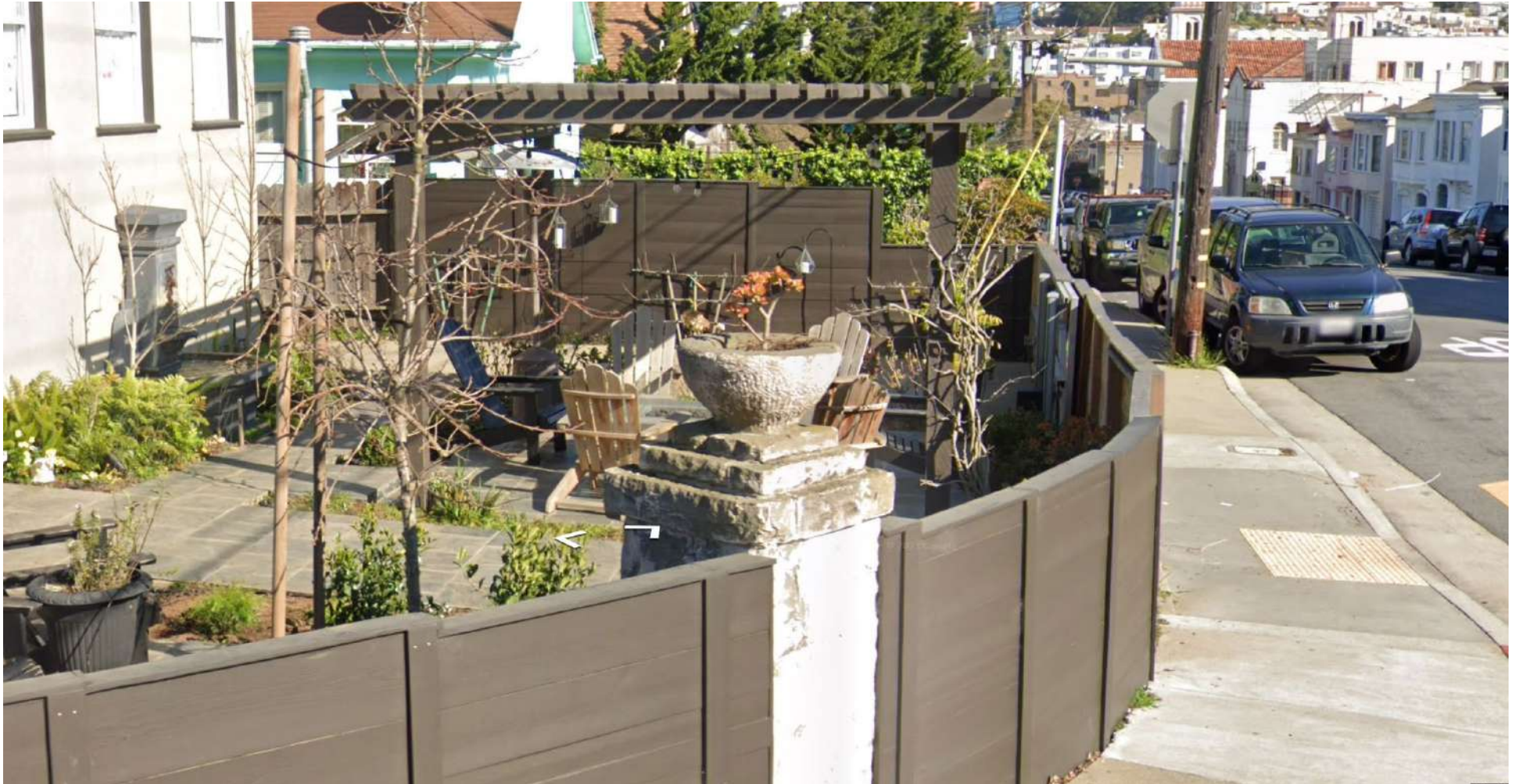
Portions of the pergola, gas fire table, landscaping, special pavers, and fence encroaching onto Ashton Ave.
