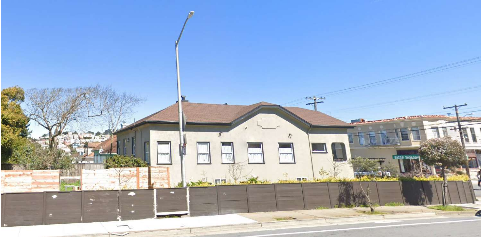
Access to PUC streetlight is prevented by the fence along Holloway Ave. Fence encroaches approximately nine feet into the right-of-way.
