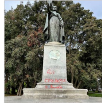
Figure 31: Detail of graffiti tags on the granite pedestal before treatment.
