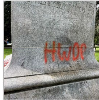
Figure 30: Detail of graffiti tags on the granite pedestal before treatment.
