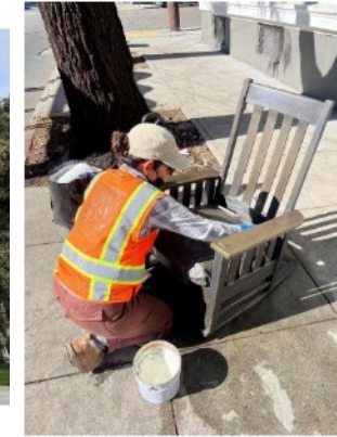
Figure 5: Conservator applying microcrystalline wax after cleaning the bronze chairs.
