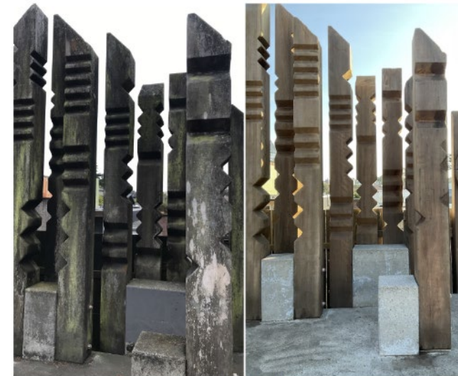
West End Before (Left) and After (Right) Treatment
