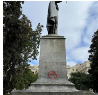
Figure 30: Detail of graffiti tags on the granite pedestal before treatment.
