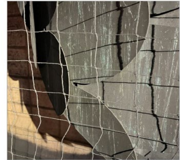
Image 6: Detail of the scales. Overall, it appears that the scales are well attached, ARG/CS January 2023.
