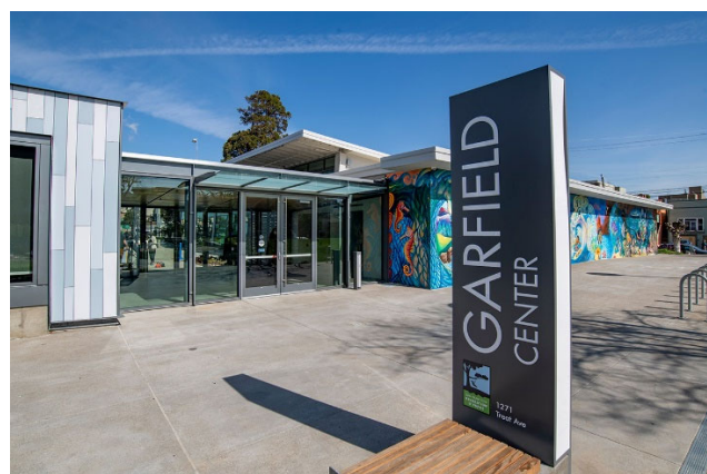
Project Complete, April 2021
