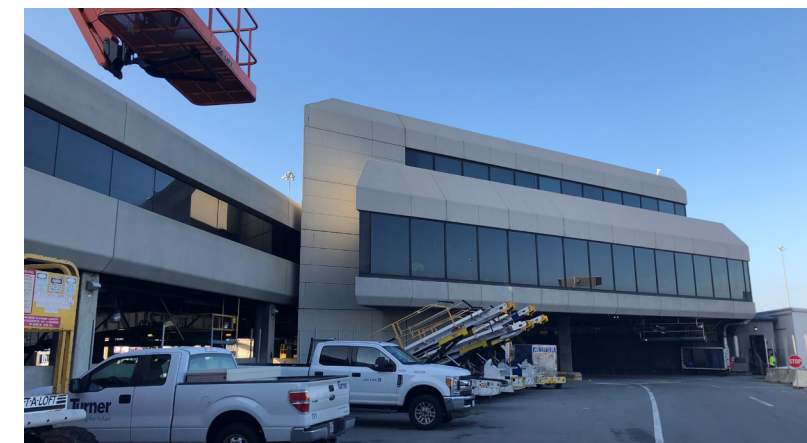
C. EXISTING STATIONS OPERATIONS CENTER
