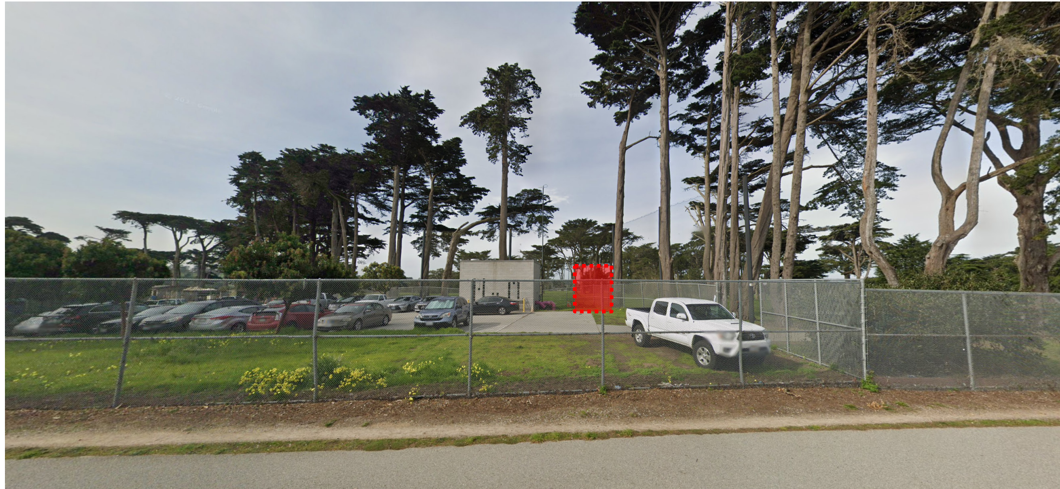
VIEW OF EXISTING PUMP STATION FROM LAKE MERCED BLVD.
