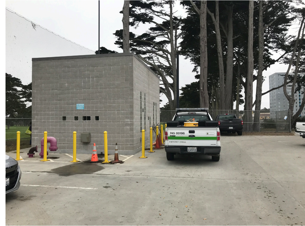
EXISTING PUMP STATION
