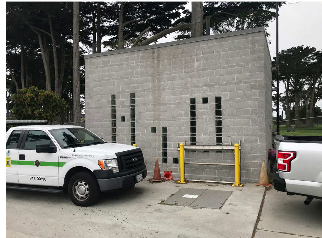
EXISTING PUMP STATION
