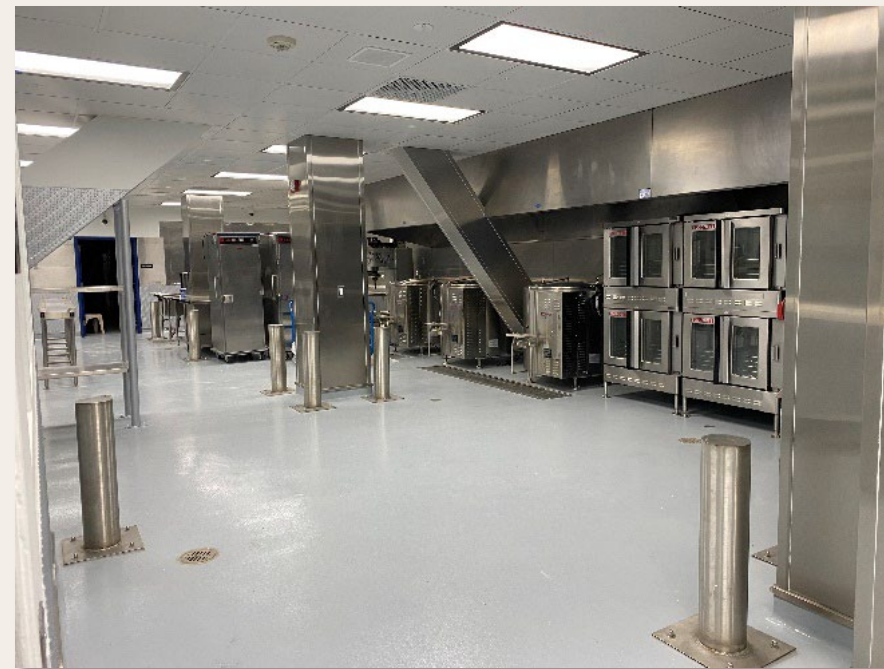
Kitchen Remodel: Capital project incarcerated person kitchen
