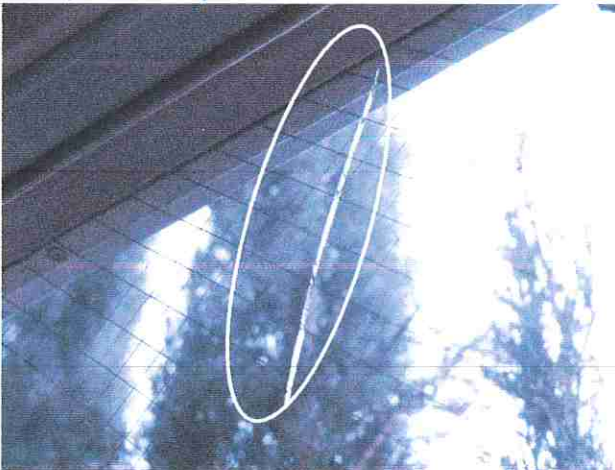
Living room Window cracked by Votrubas nailing boards to window nailing boards to the windows
