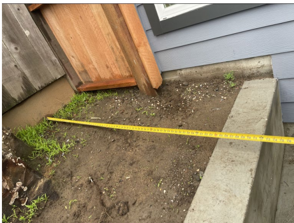
The concrete retaining wall is approximately 5 feet 4 inches setback from the other side neighbor's property line.
