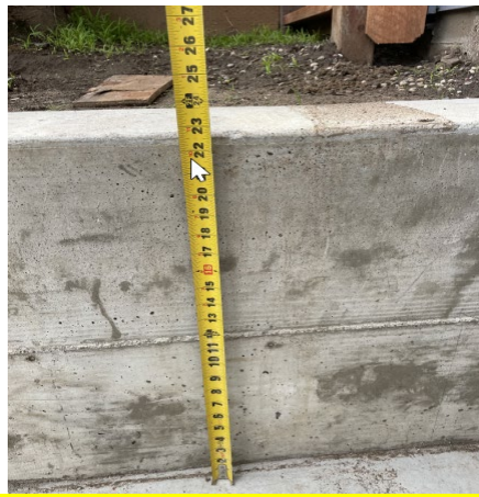
The concrete retaining wall is approximately 8.5 inches wide and the height from the inner is approximately 23 inches.
