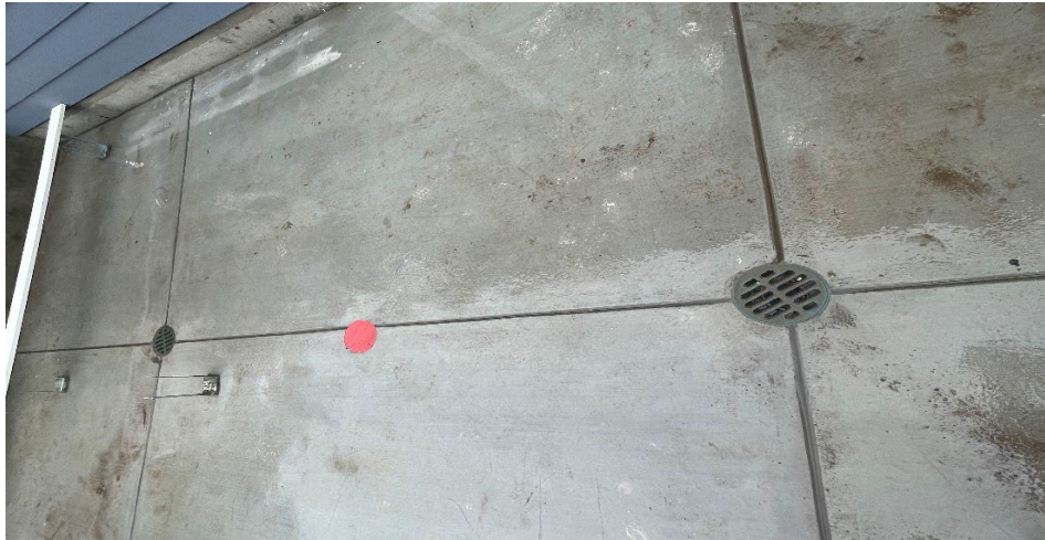
Photo of the Floor Drains
