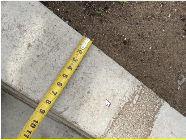
The concrete retaining wall is approximately 8.5 inches wide and the height from the inner is approximately 23 inches.
