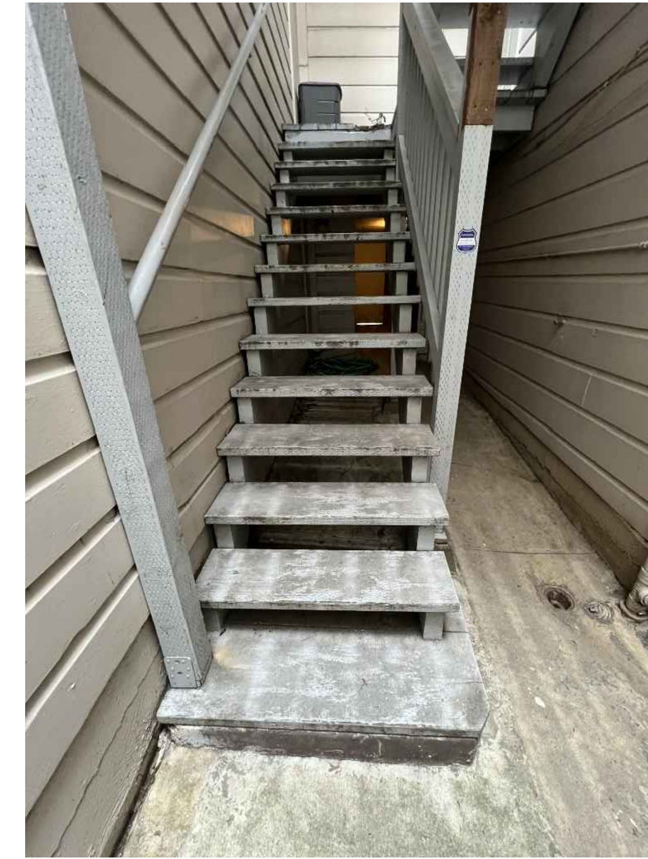
3 (E) STAIRS FROM GROUND LEVEL TO 2ND FLR
