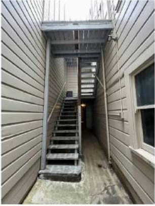
1 (E) FIRE EGRESS STAIRS
