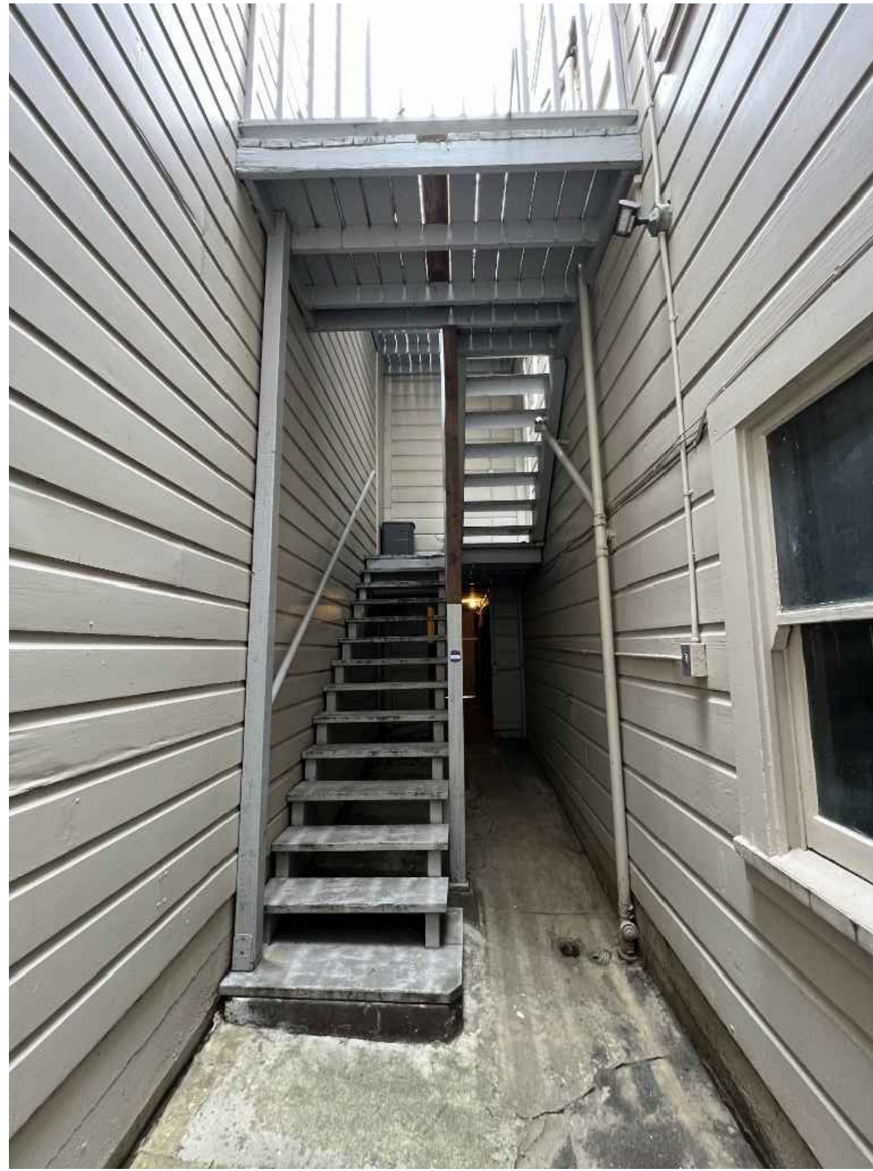
1 (E) FIRE EGRESS STAIRS
