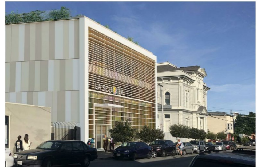
3270 18th Street expansion beside the existing building at 3250 18th Street, rendering by Perkins&Will and ZPZ Partners
