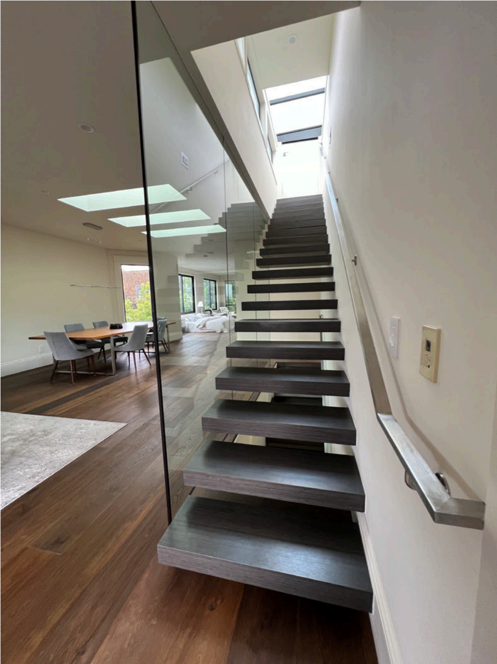
Interior Cantilever Stairs:
