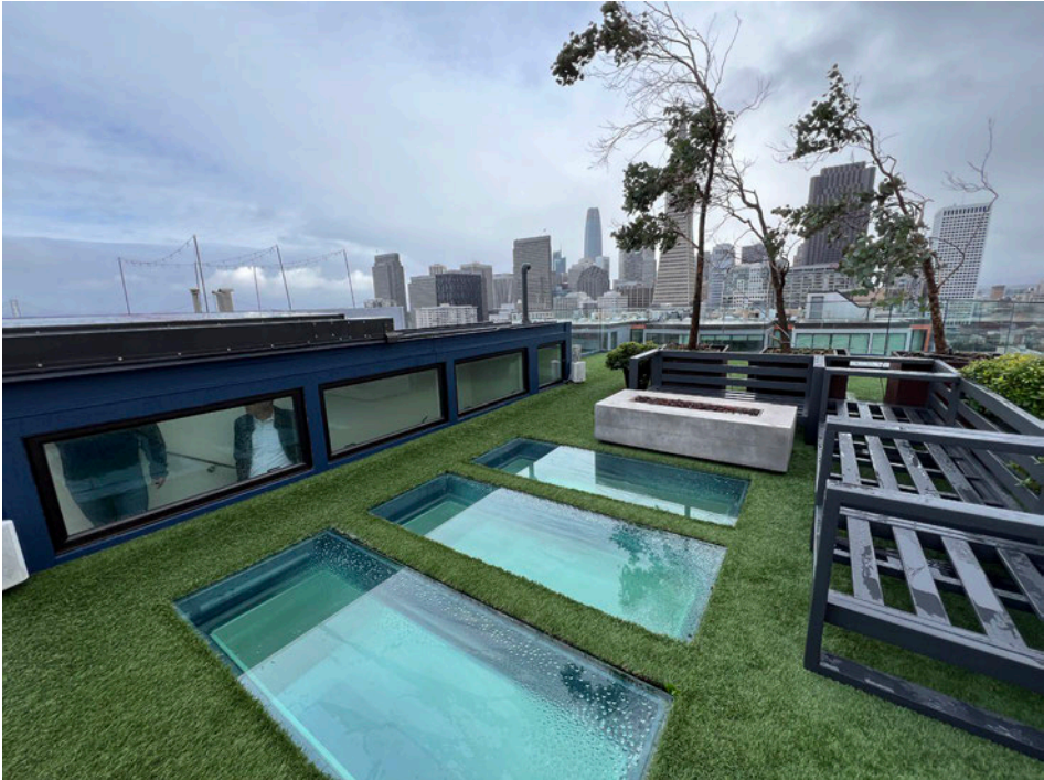
Three Stairwell Windows Installed ITEM #5:
