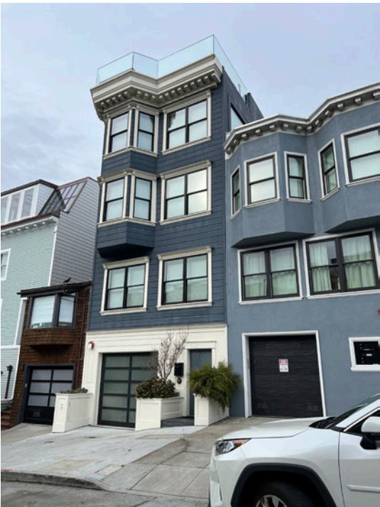
Front Garage Façade and Garage Door: (ITEM #3)
