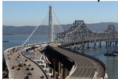
Bay Bridge Rebuild
