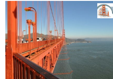
Golden Gate Bridge Suicide Deterrent Net System
