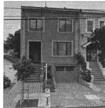
AS BUILT SITE CONDITION PHOTOGRAPH SCALE: NTS
