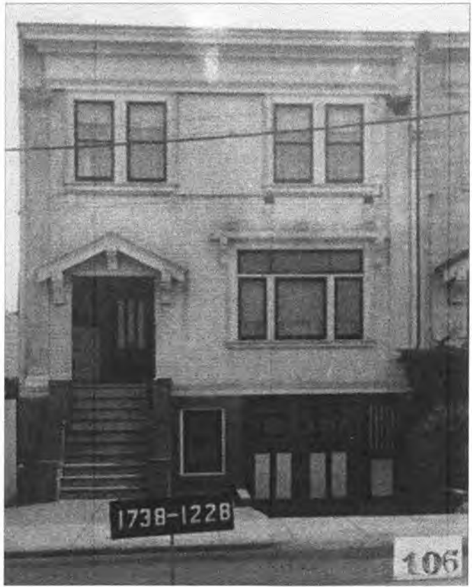
ARCHIVAL PHOTOGRAPH OF ORIGINAL EXISTING CONDITION SCALE: NTS
