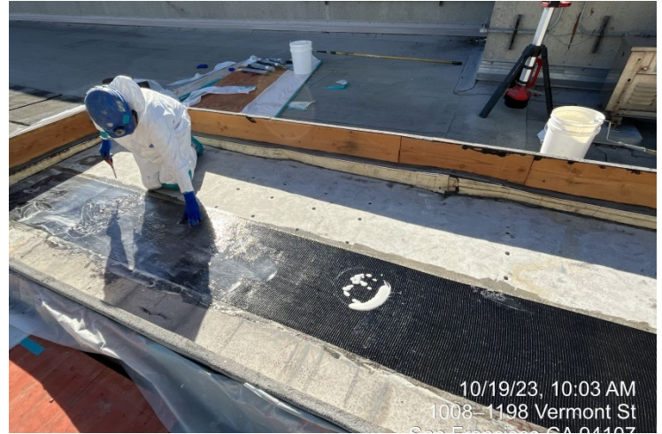
FRP Horizontal Installation at Roof Level Slab
