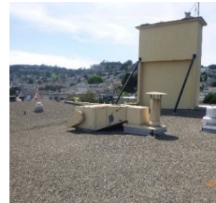
Fire Station Hose Tower
