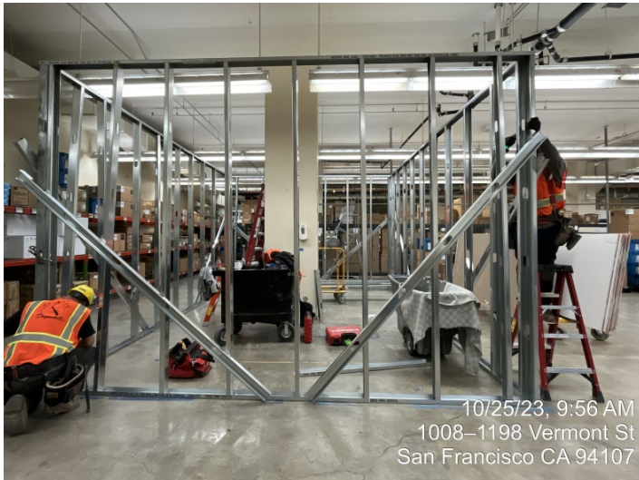
Metal Framing Installation for Infection Control Barrier at Ground Flr
