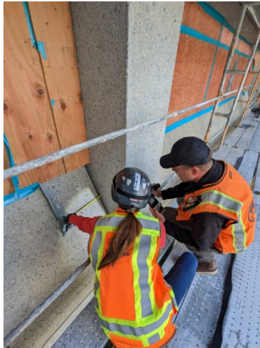
Exterior sawcutting at spandrel locations
