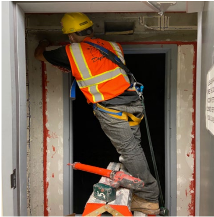
Elevator Shaft #4 Infill Framing
