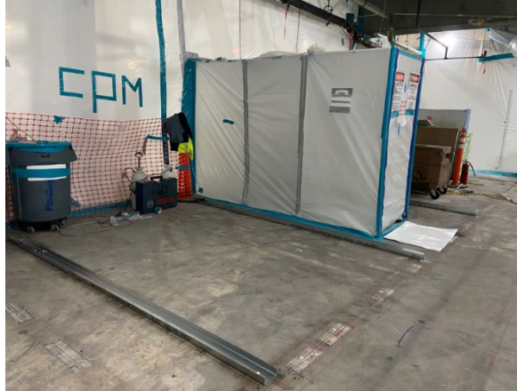
Negative Containment around Plumbing Trenching
