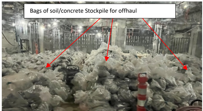
Soil/Concrete Off-haul Stockpiles at Plumbing Trench
