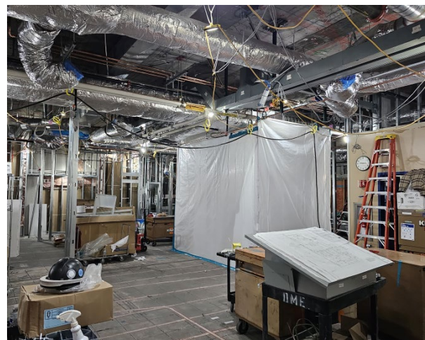
Main Space – Haz Mat abatement at column furring
