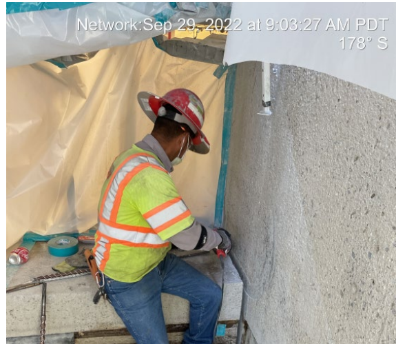
Exterior sawcutting at spandrel locations
