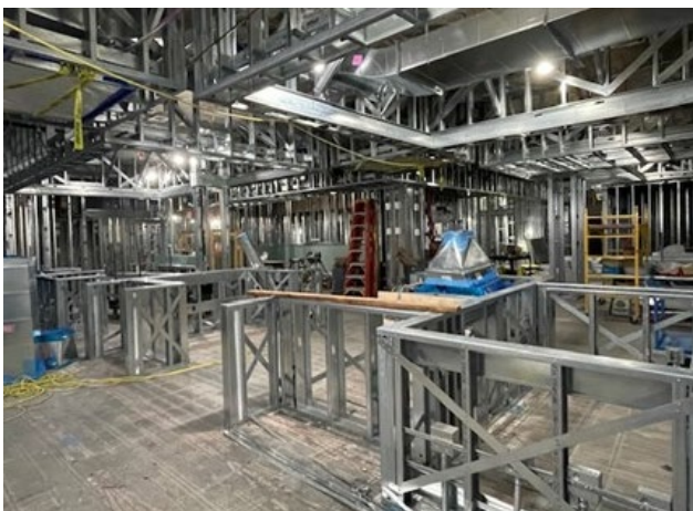
N/W Nurse Station/Treatment Bay Framing
