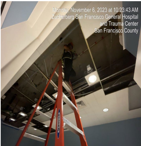
L2 North Dining – Ceiling Concrete Slab Scanning
