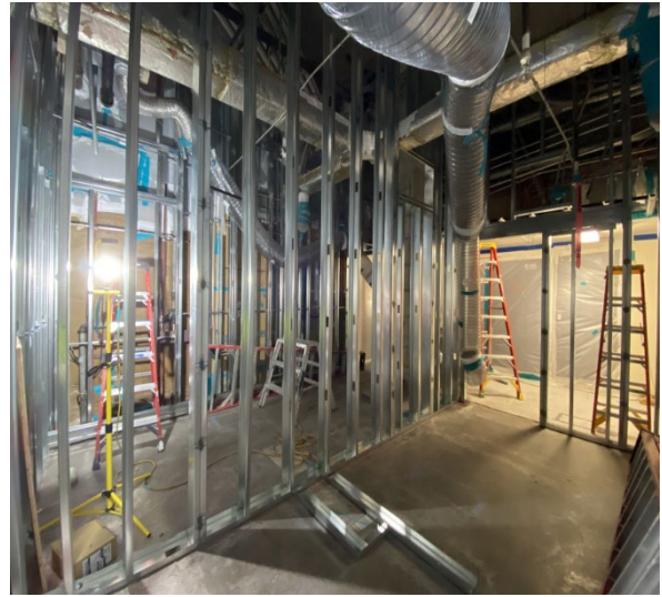
Framing in the Shower Rooms on the Ground Floor
