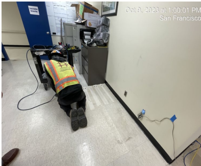
Concrete Slab Scanning in Room 2D3
