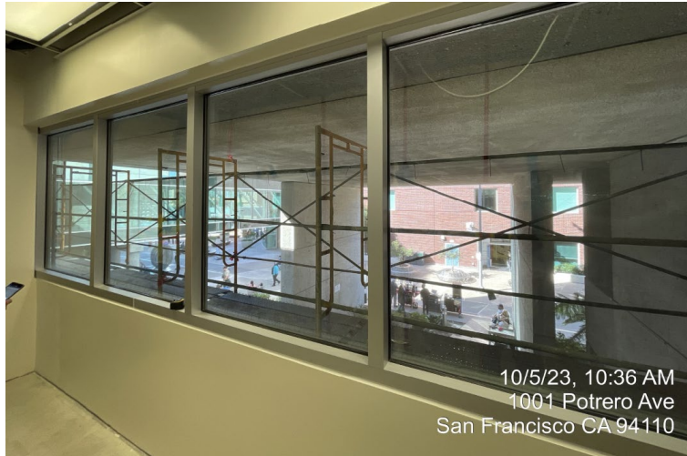
New window and interior finishes at L2 FRP Columns
