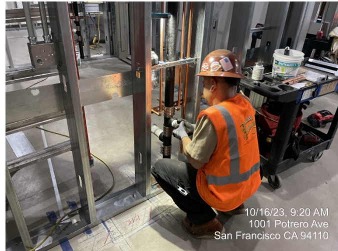
Plumbing Installation in Urology
