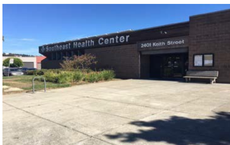
Existing SE Health Center
