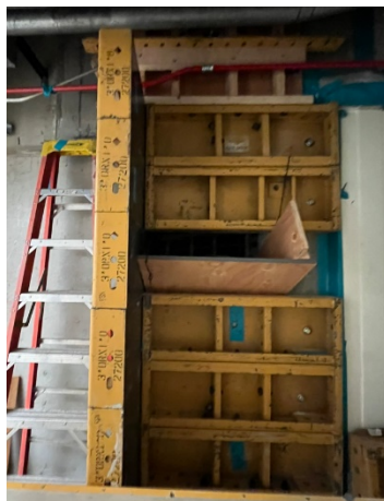
New L2 Columns for Seismic Expansion Joint between Building 5 and M-Wing
