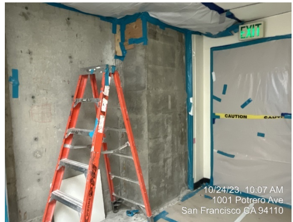
New L2 Columns for Seismic Expansion Joint between Building 5 and M-Wing
