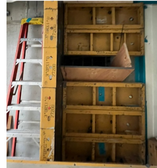
Seismic - New L2 Columns for Seismic Expansion Joint
