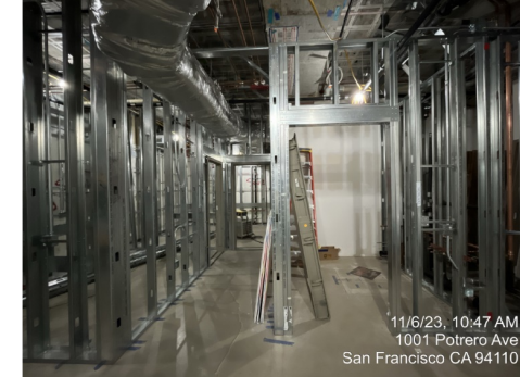
Rehab Ph 3 - Framing
