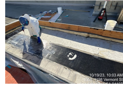
Seismic - FRP Installation at Roof Level
