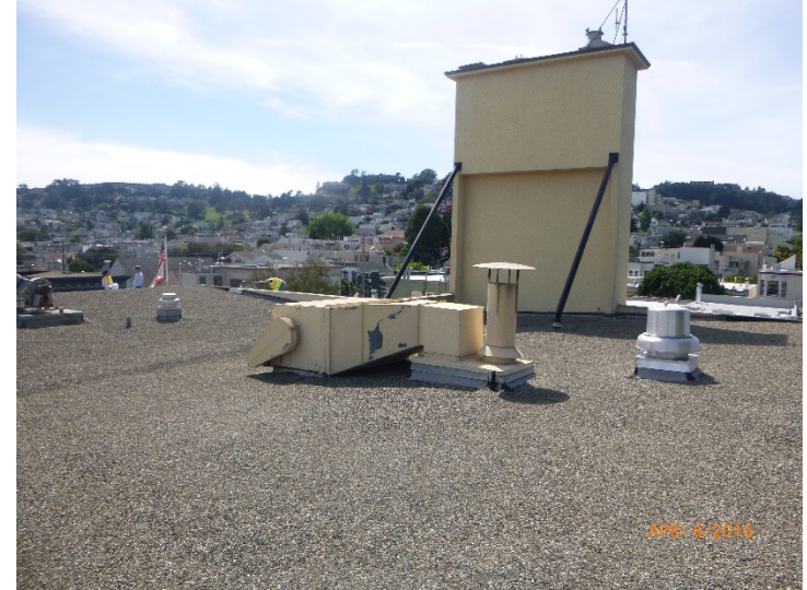
Hose Tower – Fire Station 11
