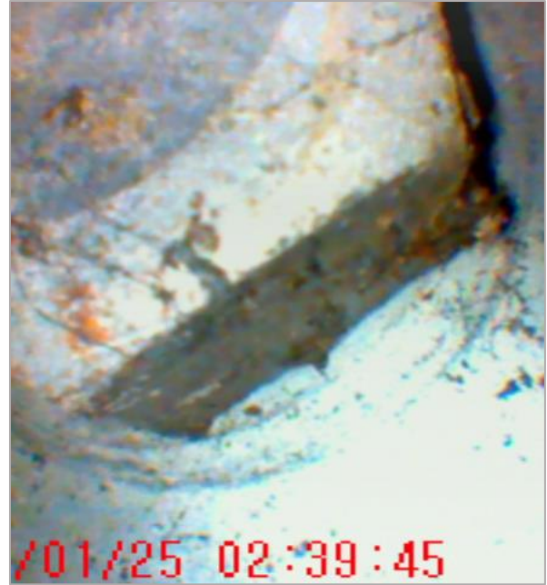
Image 10: Above is a detail of a bolt, which supports the information that the sculptures were attached to horizontal channels mounted on the building prior to the sculpture's installation, ARG/CS January 2023.
