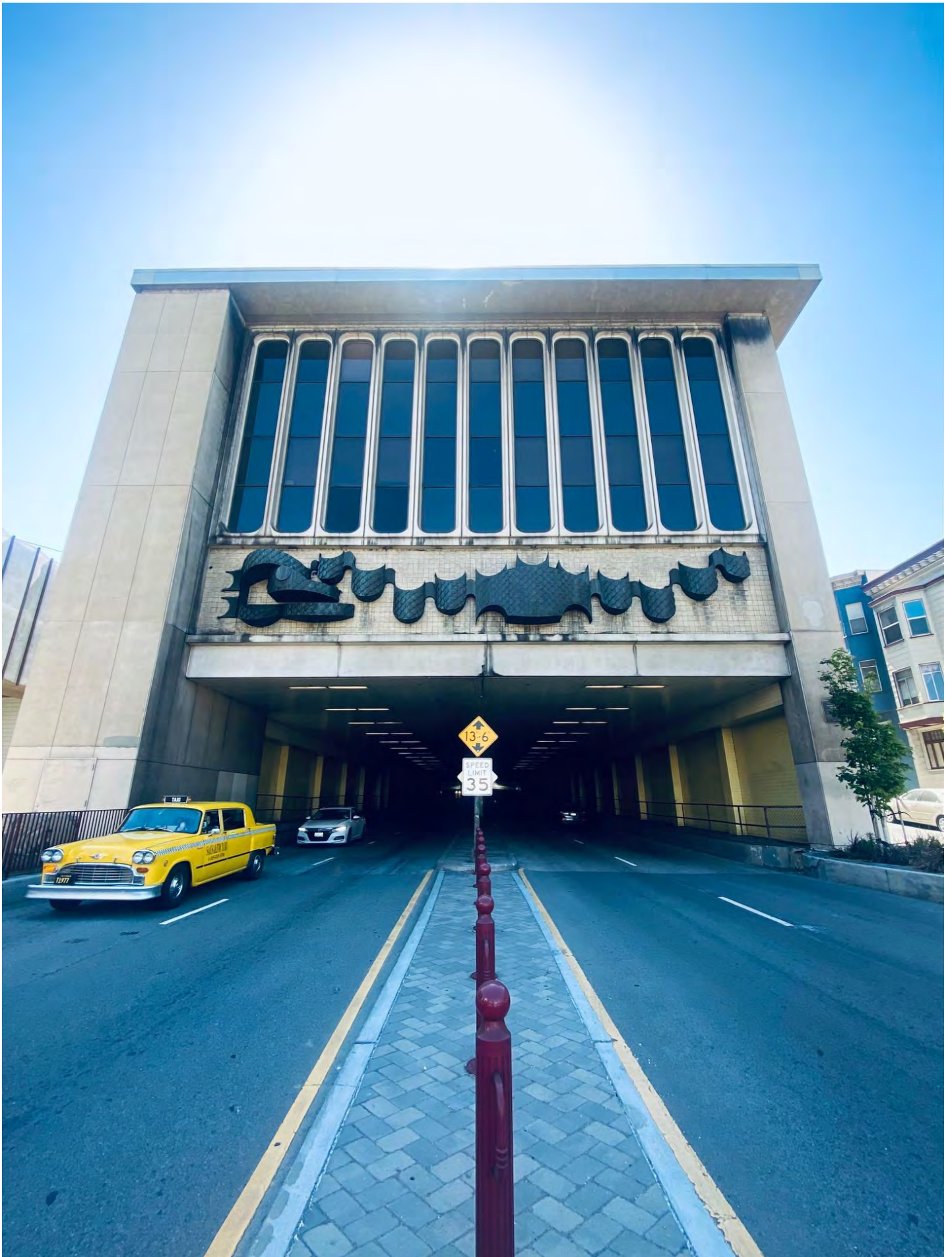
A dragon relief guards the Broadway tunnel and Chinatown Public Health Center that sits above. (Courtesy Johnny Dismal)
