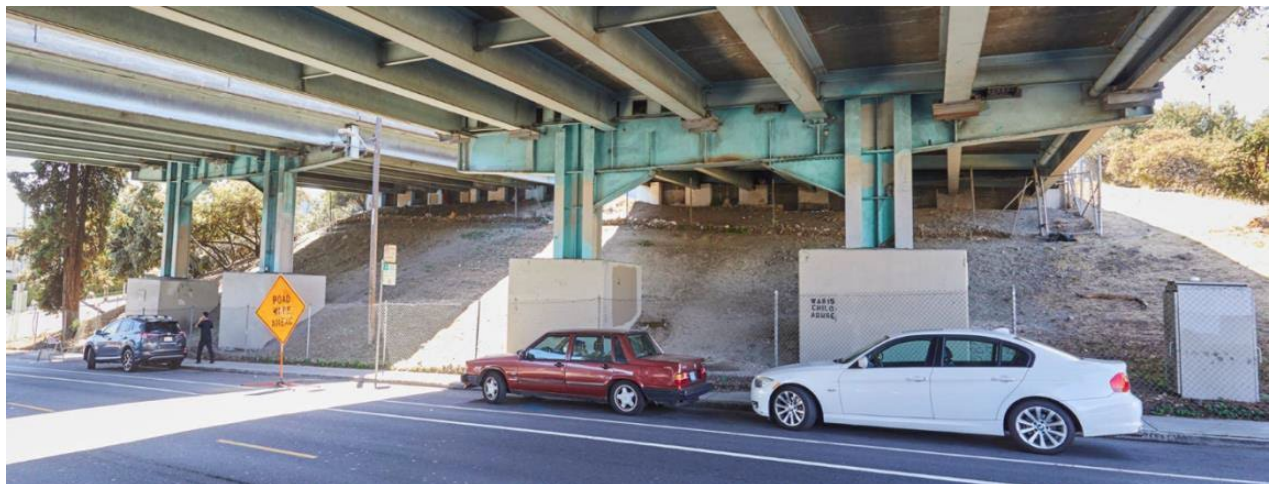
View of the Potrero Gateway Park under overpass
