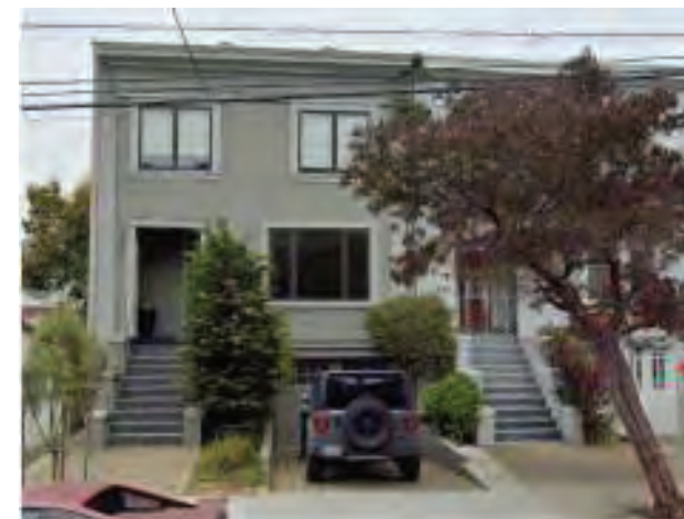
AS BUILT FACADE
