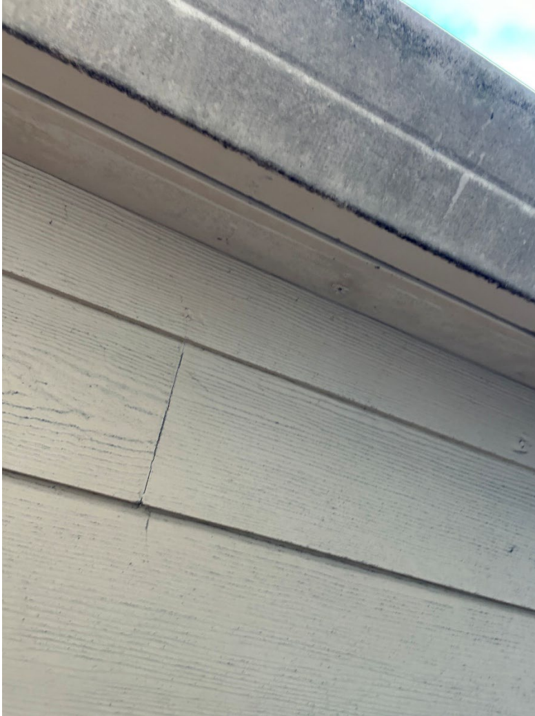
View from 225 Anderson's st. kitchen window, looking up – equivalent to leaning on the window on the inside.
