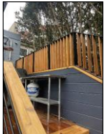
LOUVERED WOOD SLATS AT TOP 2' OF FENCE
