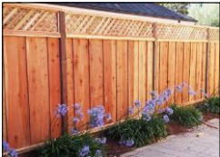
LATTICE TOP AT TOP 2' OF FENCE
