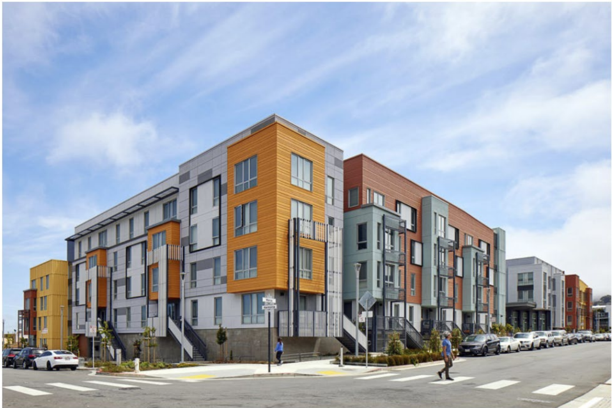
Sunnydale Block 6 (photo by Bruce Damonte)
