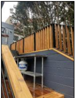
LOUVERED WOOD SLATS AT TOP 2' OF FENCE
