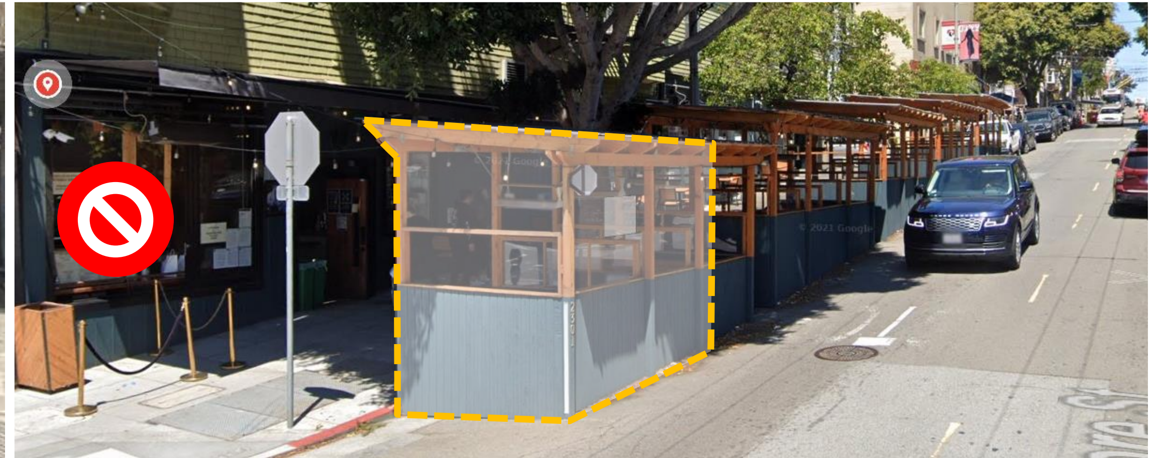
Difficult for pedestrians to see oncoming cars
