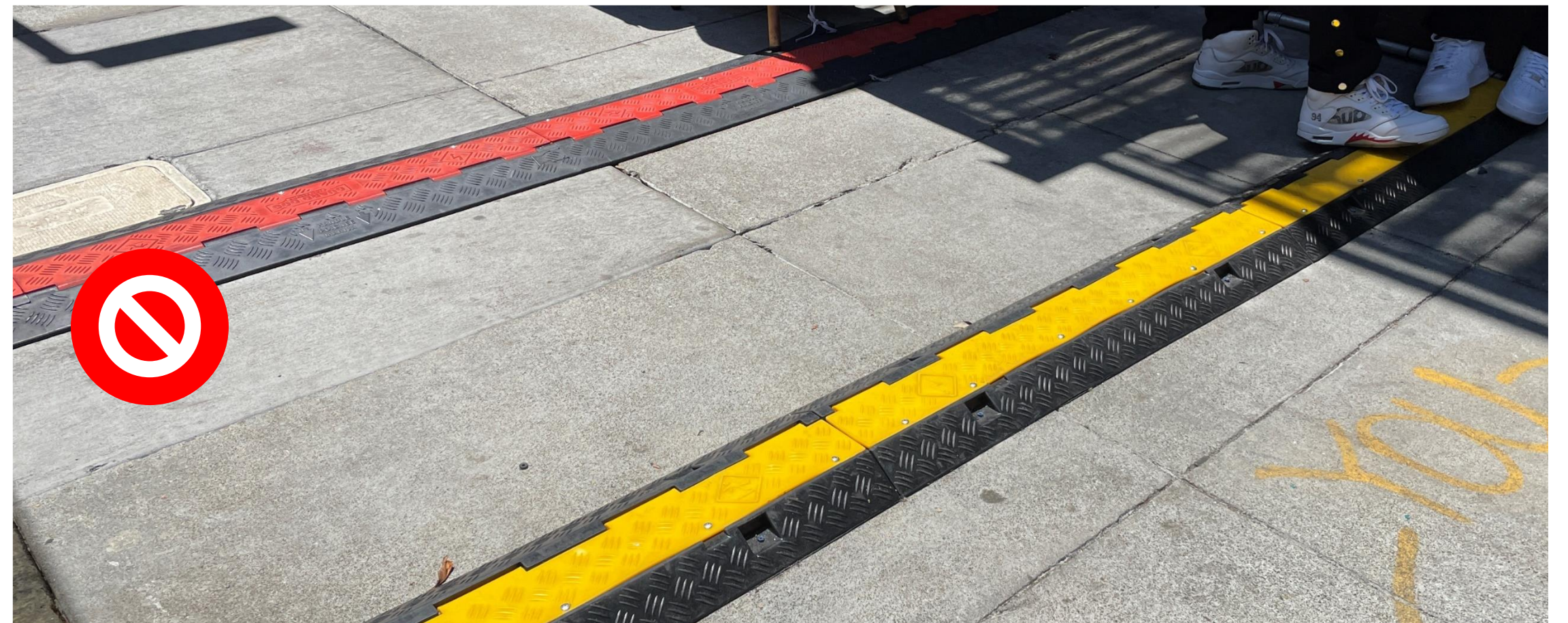
Cable ramps are bad for wheelchairs
