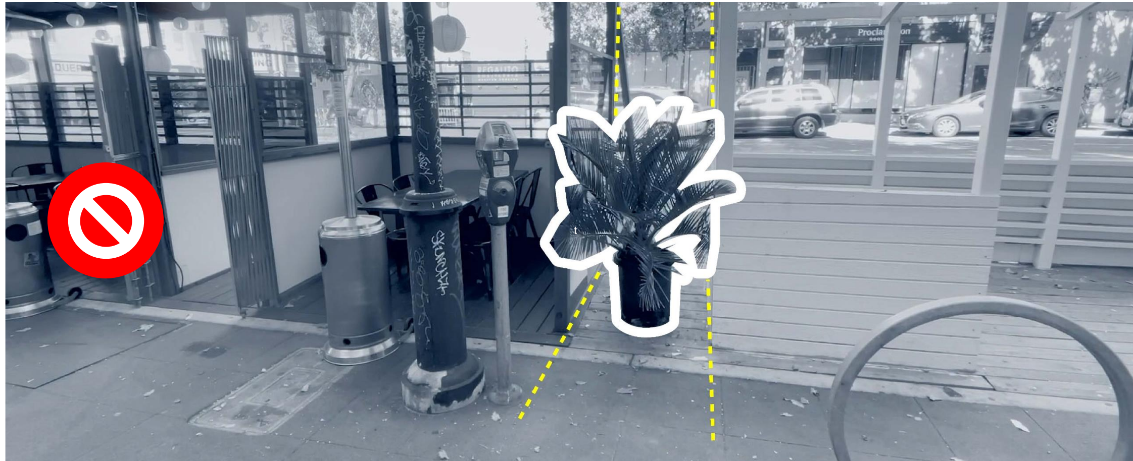
plant in path of travel
