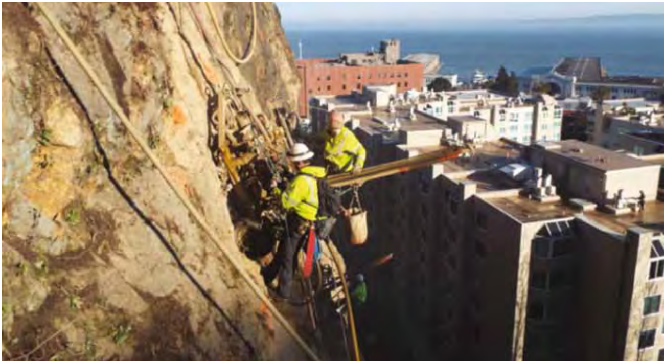
Telegraph Hill stabilization.
