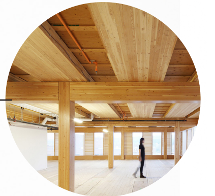
CLT & GLULAM STRUCTURE (DOUGLAS FIR)
