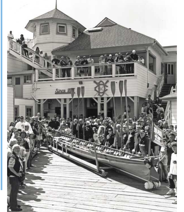
1997 Weiland Restoration Launching
