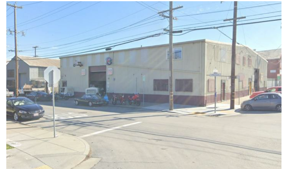
C East Corner of Phelps-Jerrold Intersection
