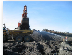
Article 31 applies at The Shipyard for large earth moving projects
