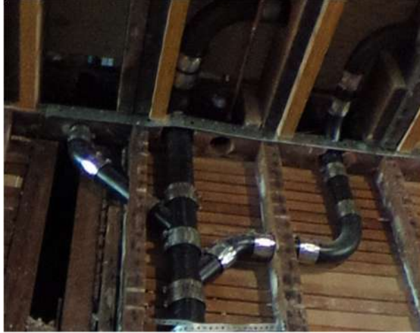
Photo 1: New Drain Lines installed in Shared Property Line Bearing Wall
