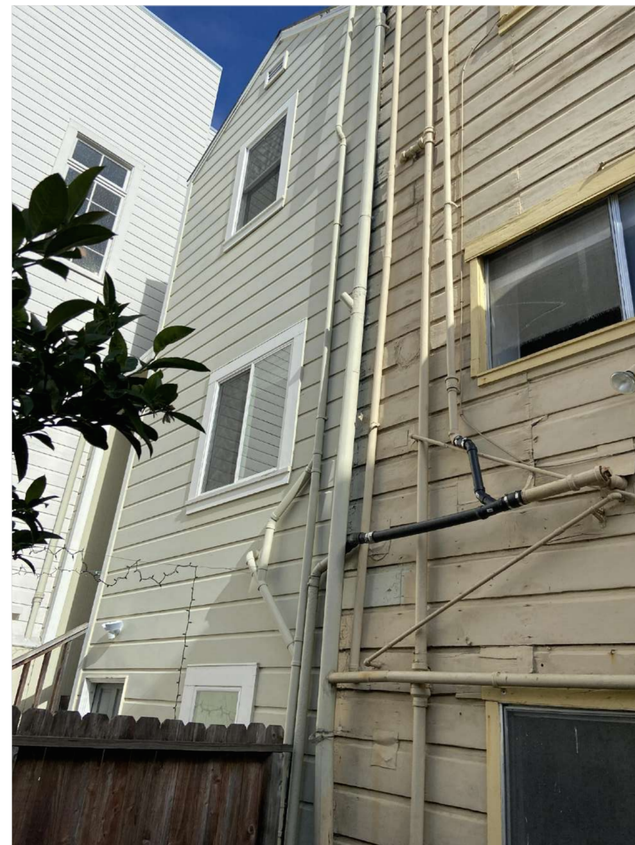
4 ADJACENT PROPERTY ON WEST
