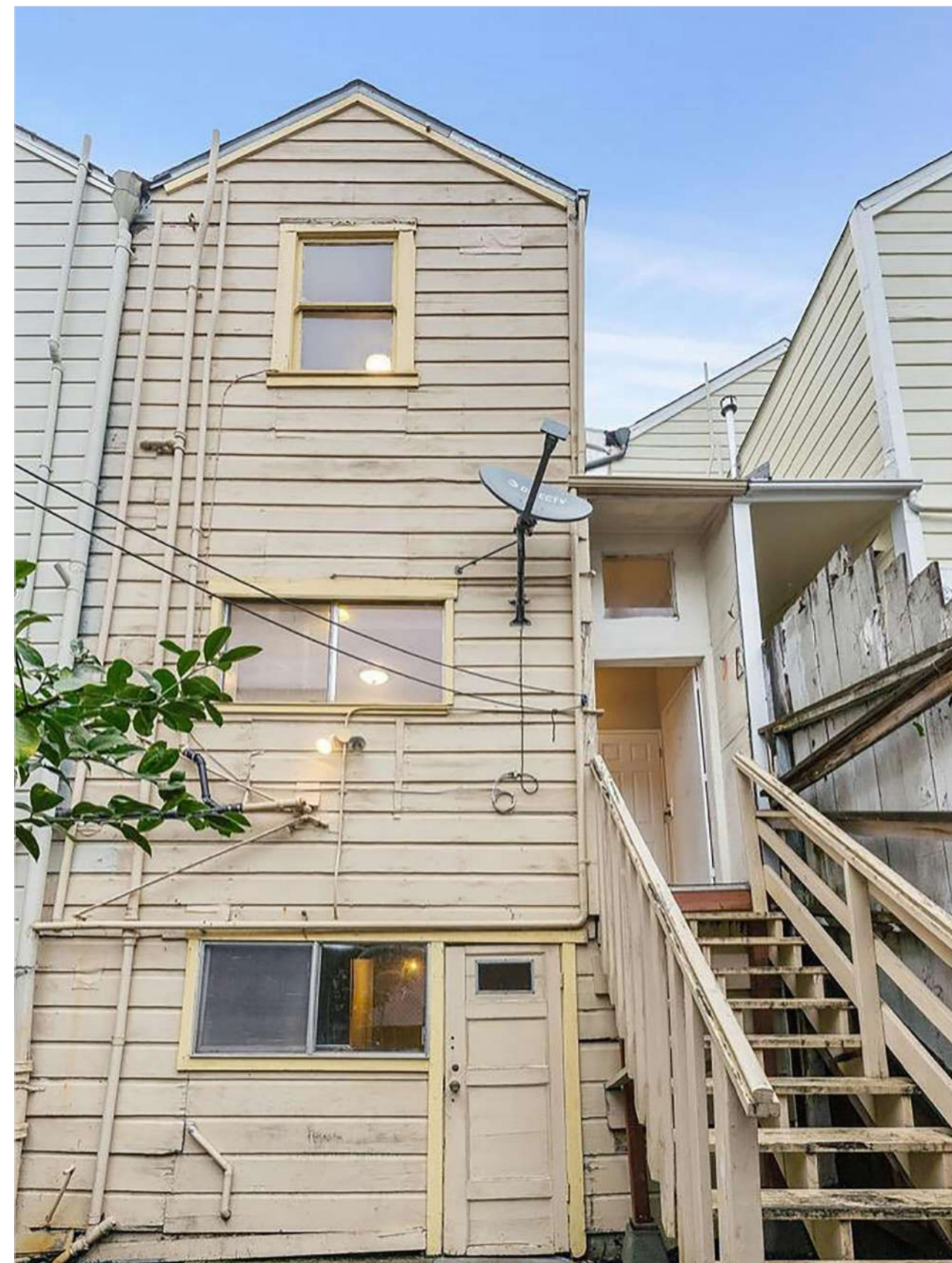
1 REAR FACADE AND ADJACENT PROPERTY EAST
