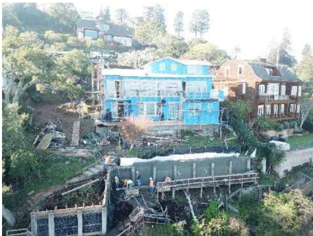
312 Beach Road, Belvedere, CA Project Type: Residential Construction Design of retaining walls, landscape features, and ADU on a steep site in Belvedere.
