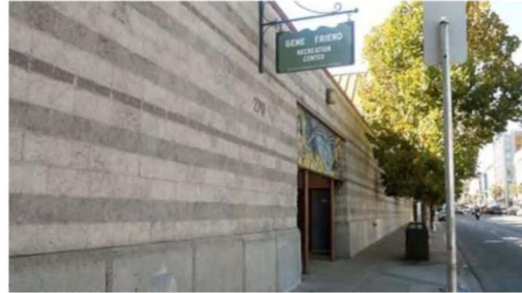
EXISTING - 6 TH STREET ENTRANCE
