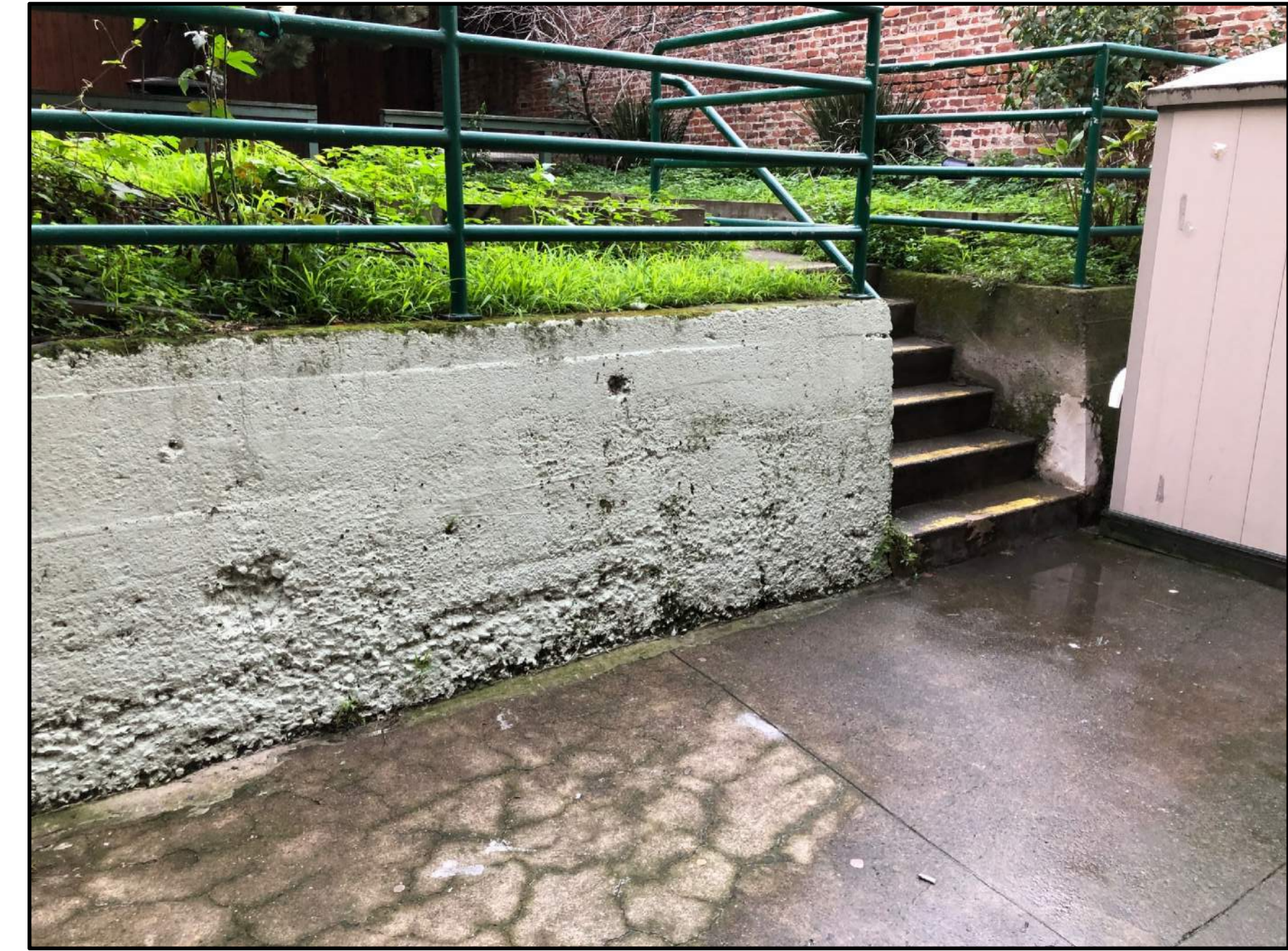
NORTH - REAR YARD
