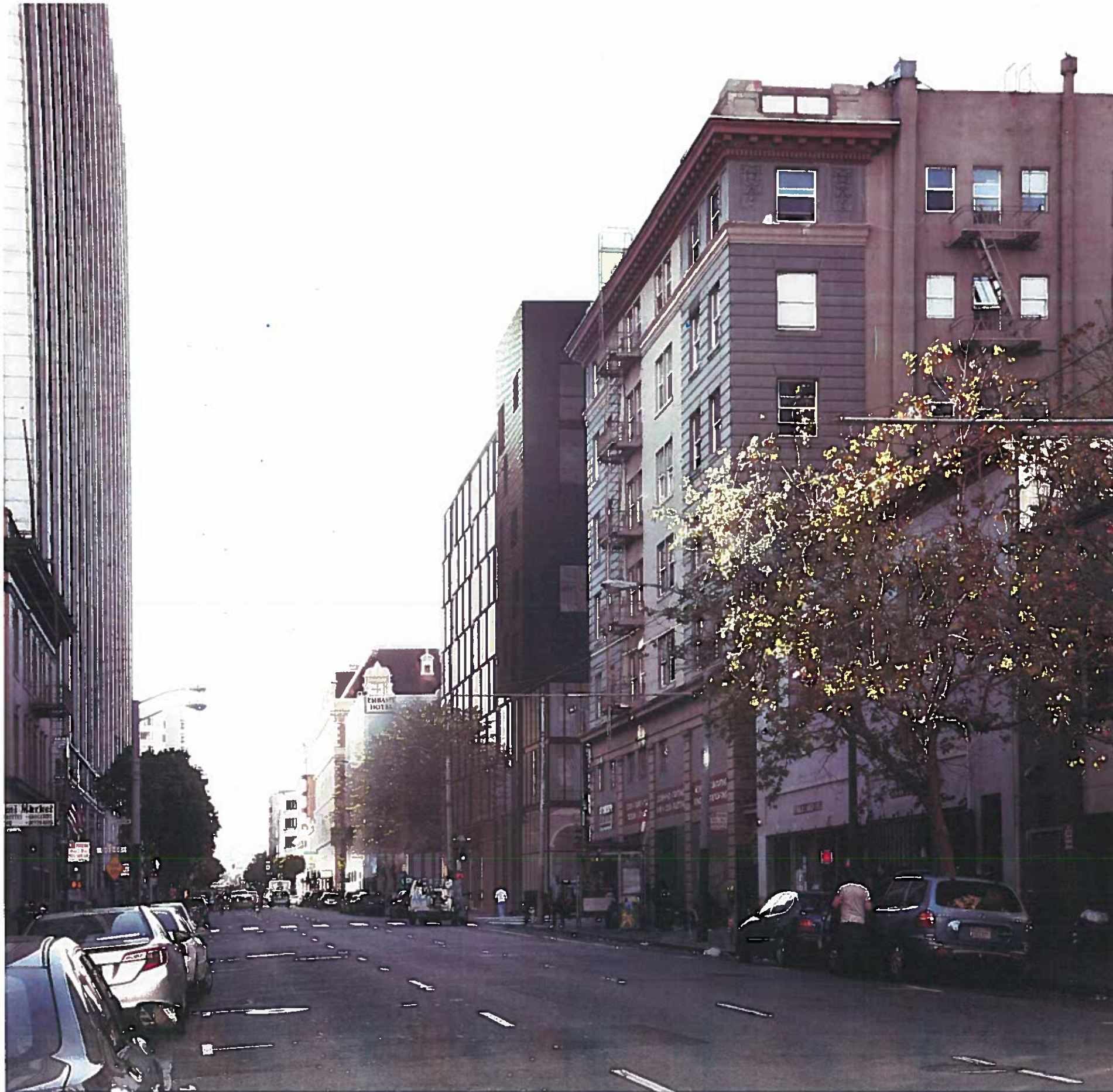
VIEW FROM LARKIN STREET LOOKING WEST (SEE FINISH SCHEDULE FOR REVISED COLORS)
