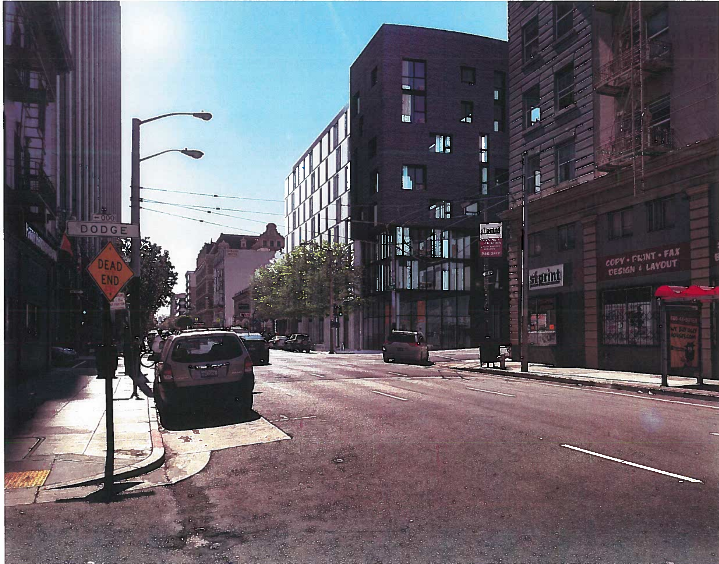
VIEW FROM LARKIN STREET LOOKING WEST (SEE FINISH SCHEDULE FOR REVISED COLORS)
