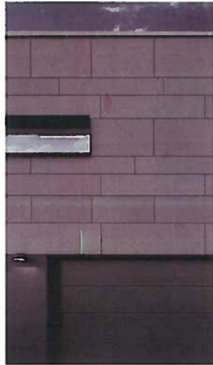
PRE-FINISHED FIBER CEMENT RAINSCREEN PANELS
