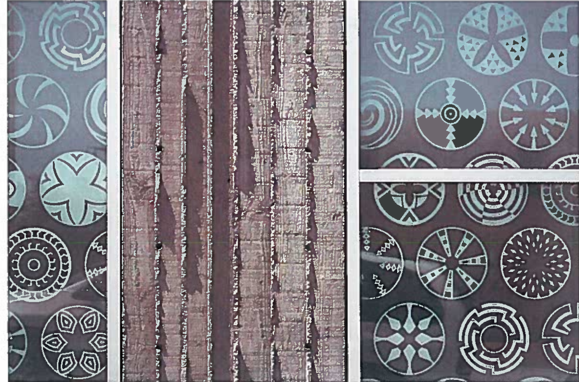
ALUMINUM STOREFRONT WINDOWS AND BOARD FORMED TEXTURED CONCRETE
